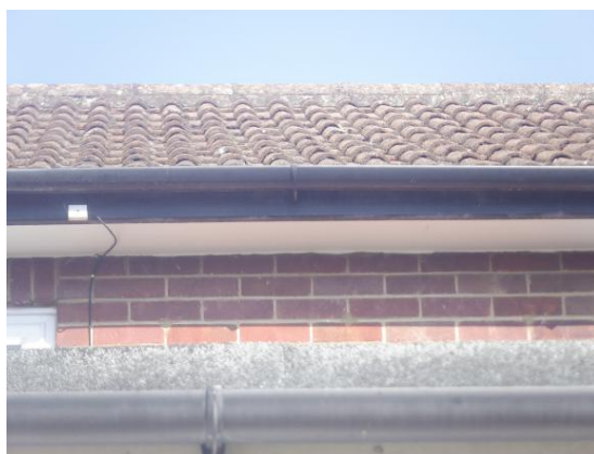
Photograph 4. Fully intact ridge mortar (rear elevation).
