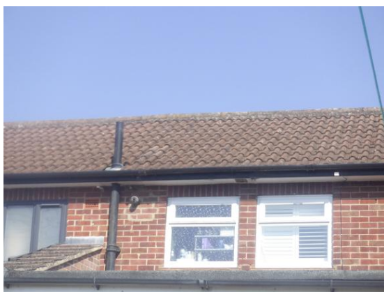
Photograph 3. Fully sealed interlocking concrete tiles (rear elevation).
