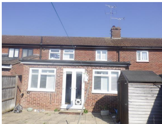
Photograph 2. Rear elevation viewed from the southeast.
