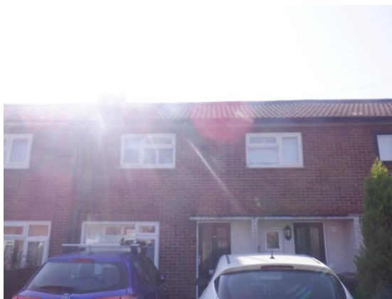
Photograph 1. Front elevation viewed from the northwest.
