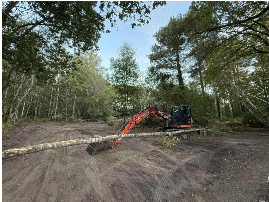
Figure 10: Photo showing clearance activities at the Range Road location of application 260439, also previously known as "The Fords". This shows the use of mechanised machinery within RPAs, strictly prohibited in the later-produced Tree Survey & Arboriculture Impact Assessment (BS5837:2012). Photo has meta-data showing location and date taken on the 25 th September 2025 at 21:05 and is unmodified from the original taken with iPhone.
