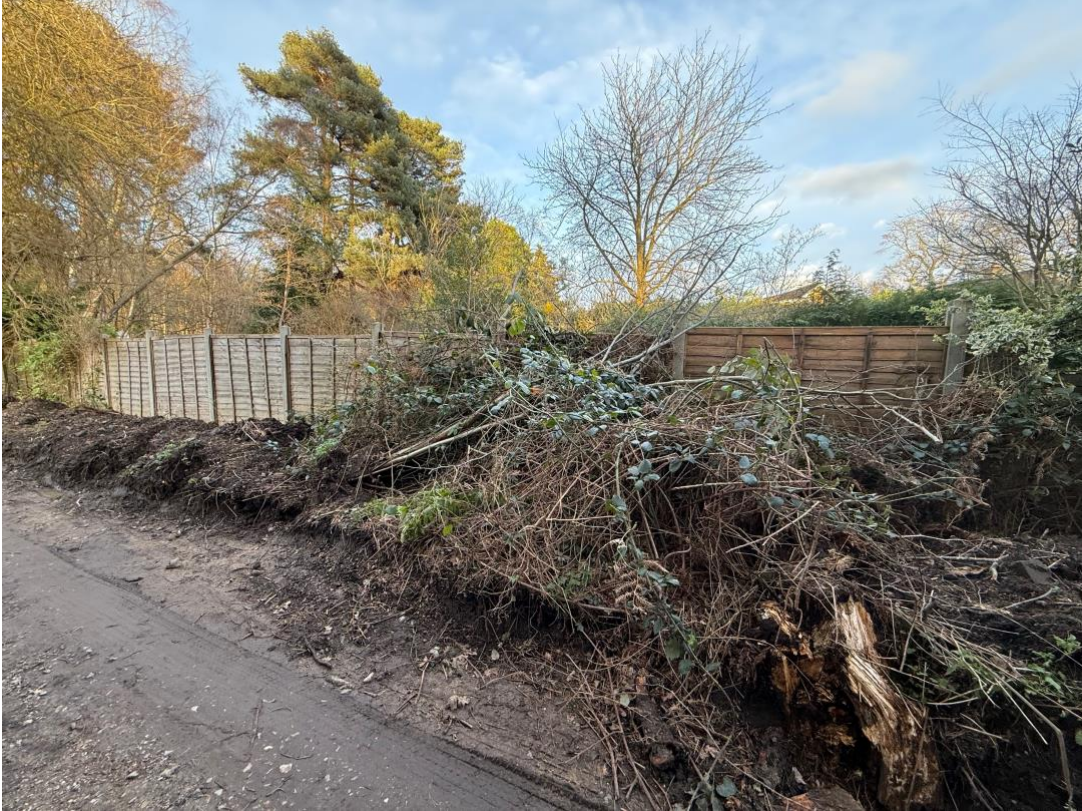
Figure 1: Showing extent of damage adjacent to property on corner of NMR and Range Road. This was deemed as “no identified damage” by the WBC PRoW Highways Team – email Tuesday 31 st March – Laura Buck) showing trees banked up against fenced boundaries during clearance and an attempted widening on to private property (as currently defined by WBC Highways Team). This activity was undertaken between 17:30am on Friday 6 th March and 03:30am in Saturday 7 th March. Photo has meta-data showing location and date taken on 13 th March 2026, at a time deemed safe for residents to approach.
