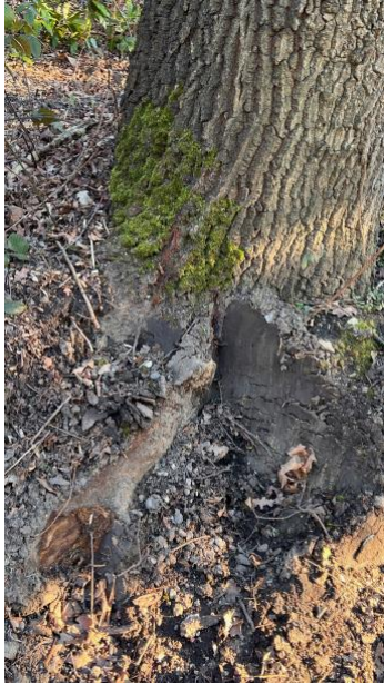
Figure 2: Showing base of oak tree and damage to root system by an attempted widening of the track with a digger at southern entrance of Range Road. By exposing and damaging the root in this way, there will be an increased risk of infection by decay pathogens. This activity was undertaken between 17:30am on Friday 6 th March and 03:30am in Saturday 7 th March, although not by the applicant for this proposed development (that I am aware). Photo has meta-data showing location and date taken on 21 st March 2026, at a time deemed safe for residents to approach.
