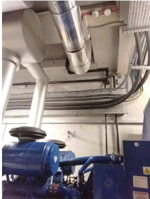
Sample of external plant areas
