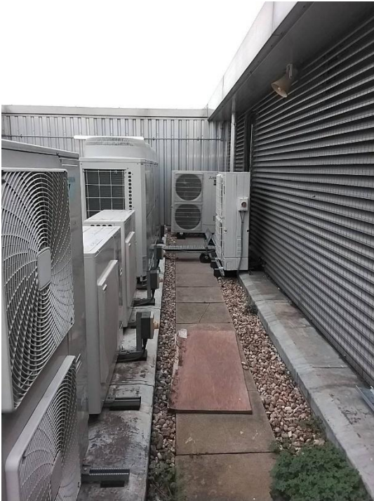
Building 1 rooftop areas
