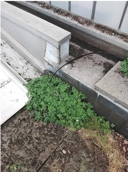
Building 1 rooftop areas
