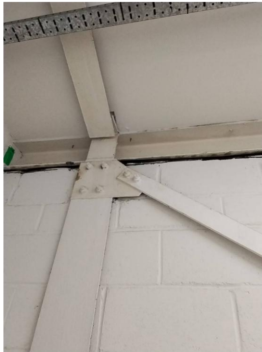
Building 1 rooftop areas
