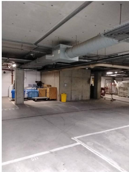
Building 1 basement car park
