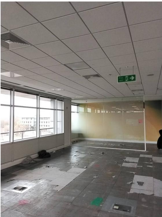
Building 2 office floors in process of strip out
