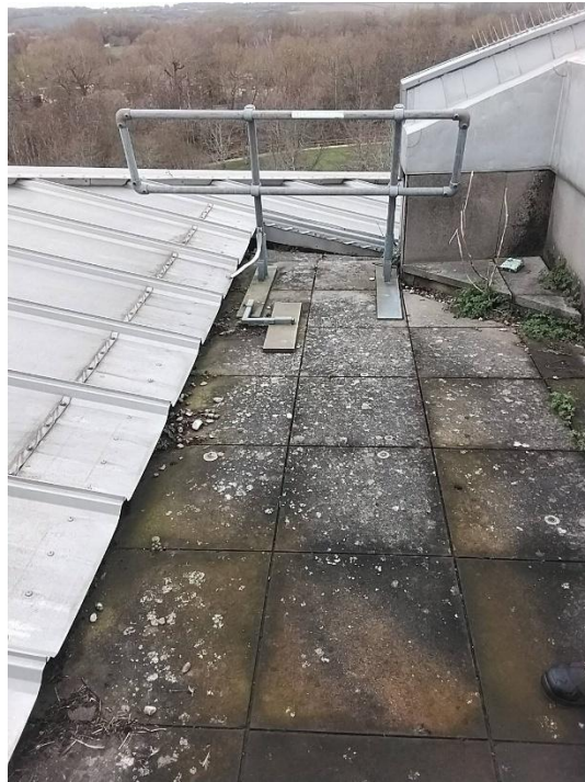
Building 1 rooftop areas
