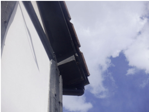
Photograph 8. Gap of limited extent behind soffit along the front gable.
