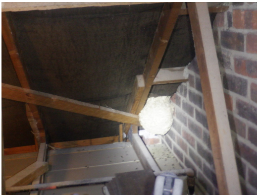
Photograph 19. Fully intact bitumen & hessian felt (Second roof void).
