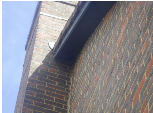
Photograph 9. Gap between timber soffit and brickwork (northwest elevation).
