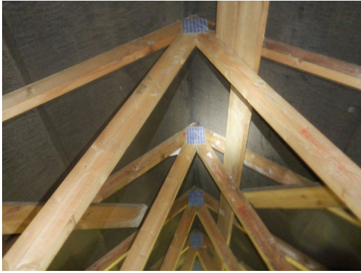
Photograph 18. Cobwebbed trussed rafters (Second roof void).
