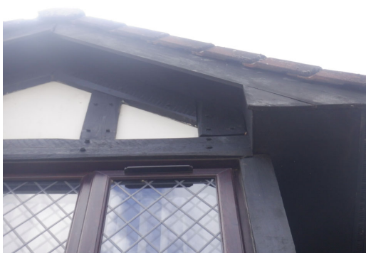
Photograph 5. Verge caps fully sealed (front elevation).
