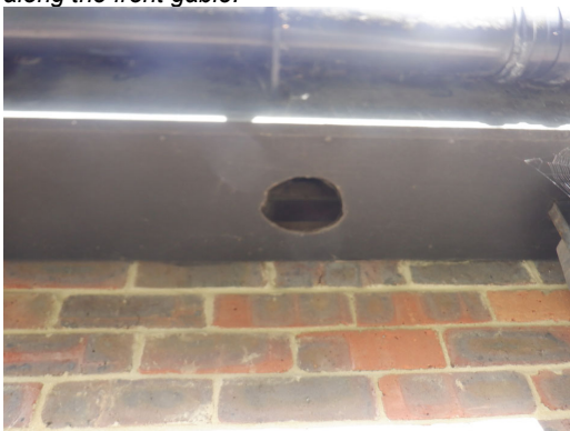
Photograph 10. Missing vent in timber soffit (rear elevation).
