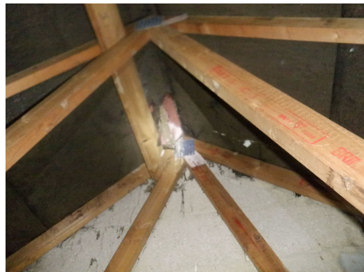
Photograph 13. Tear in roof lining along the ridge (First roof void).
