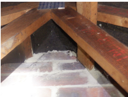
Photograph 21. Southern gable fully sealed (Second roof void).
