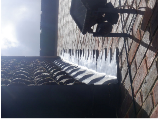
Photograph 6. Lead flashing sealed at the base of the chimney (rear elevation).
