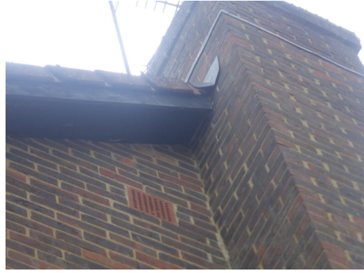
Photograph 7. Gap between lead flashing and brickwork chimney
