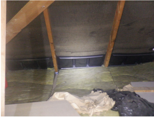
Photograph 14. Eaves blocked by plastic vent guards (First roof void).
