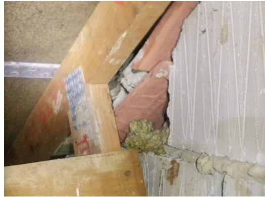
Photograph 16. Gaps along the edges of the northwest blockwork gable (First roof void).
