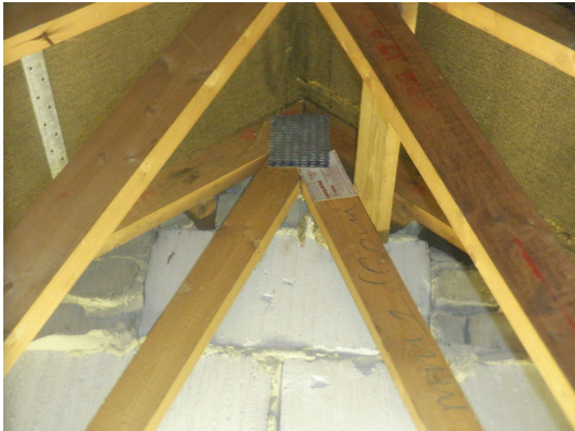
Photograph 15. Southeast blockwork gable tight to timbers (First roof void).
