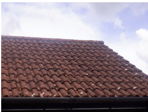
Photograph 3. Roof tiles and dry-ridge tiles flat and sealed (rear elevation).
