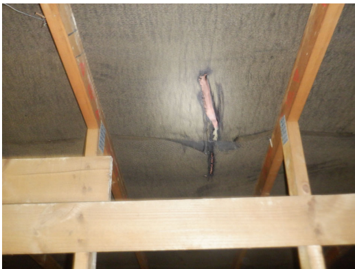
Photograph 12. Tear in roof felt (First roof void).
