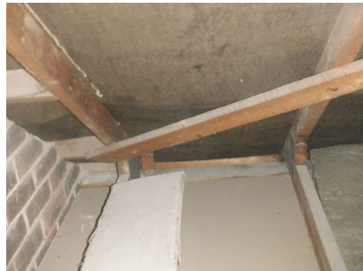
Photograph 20. Open eaves with access to the soffit (Second roof void).
