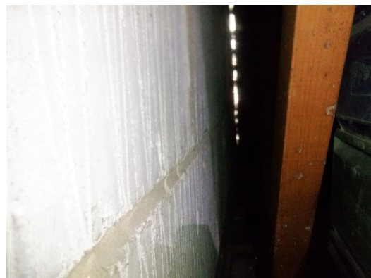
Photograph 22. Daylight visible along the edge of the northern blockwork gable (Second roof void).
