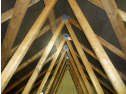
Photograph 11. Void of trussed construction (First roof void).
