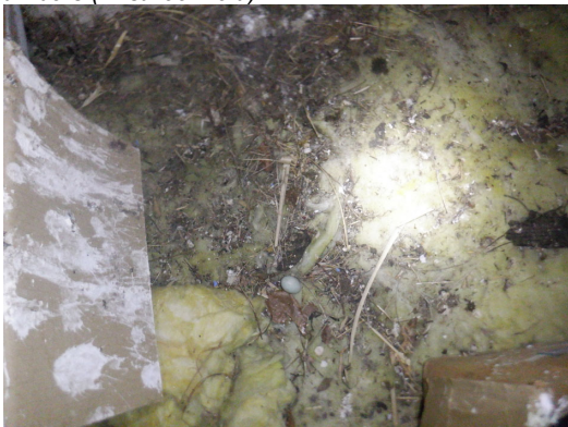
Photograph 17. Bird nesting material at the base of the northwest blockwork gable (First roof void).
