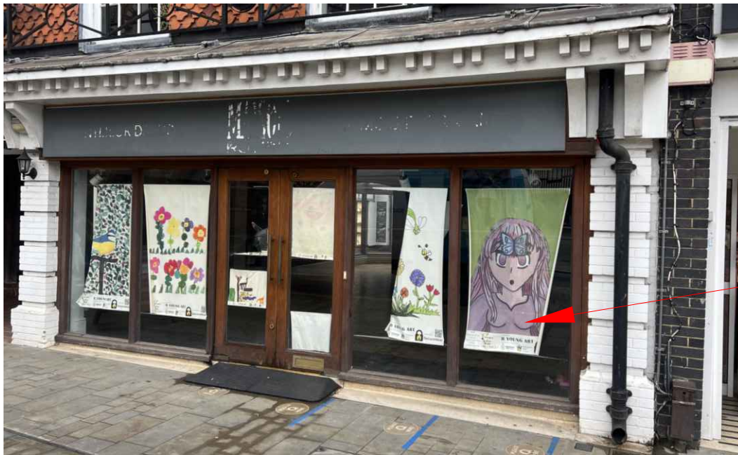
Existing shop front and window
