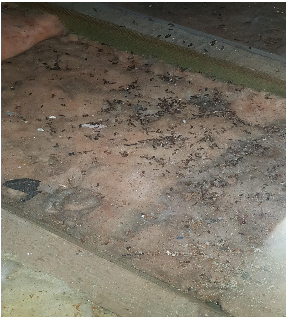
Picture 6: Showing the bat dropping on top of the insulation
