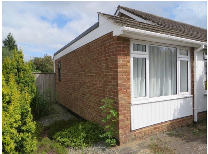
Completed front left elevation.
