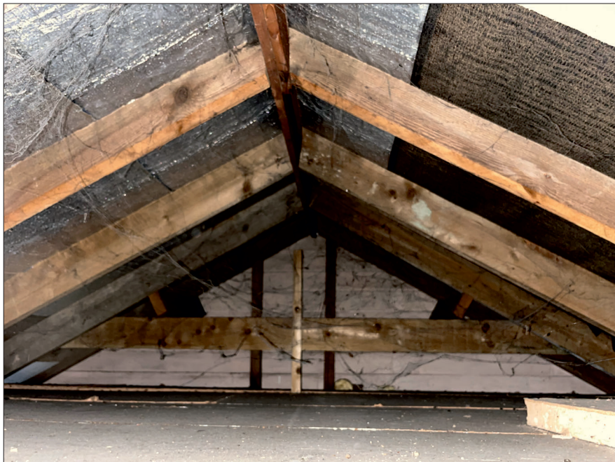
Photograph 3: Showing the restricted roof void above the rear extension.
