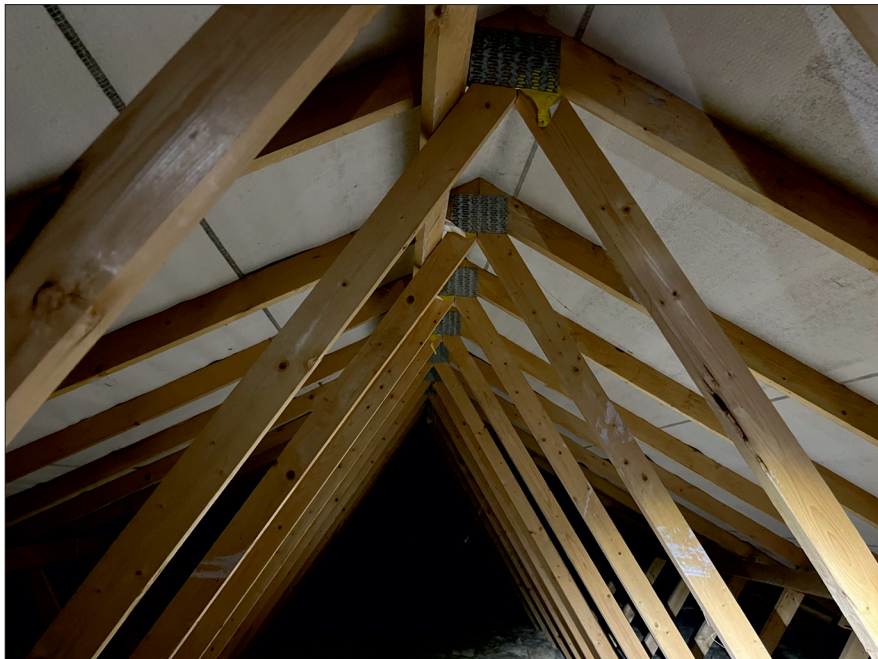
Photograph 4: Showing the main roof space/attic of the bungalow.
