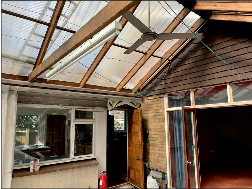
Photograph 2: Showing the internals of the rear extensions.
