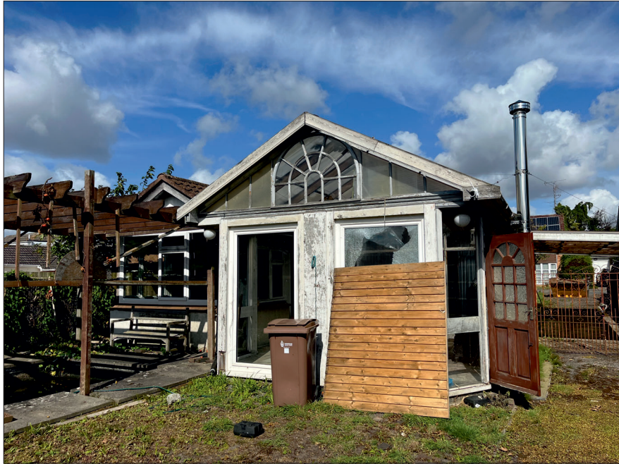
Photograph 1: Showing the rear extensions.
