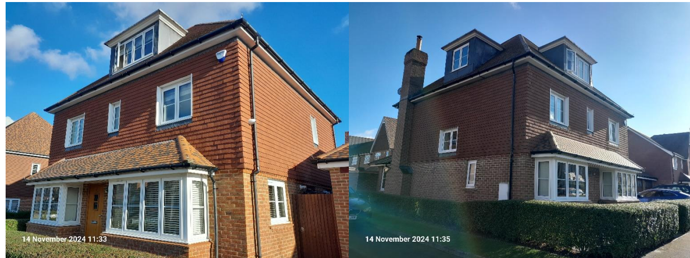
B1: southwestern elevation (left) and northwestern elevation (right).
