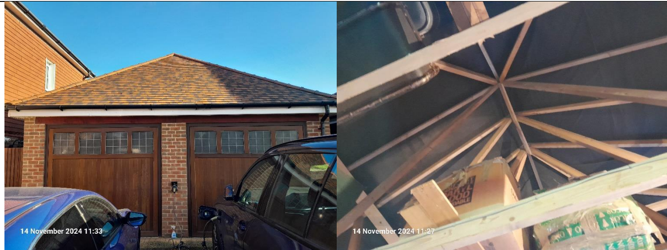
B2: the garage (left) and interior with no loft void (right).
