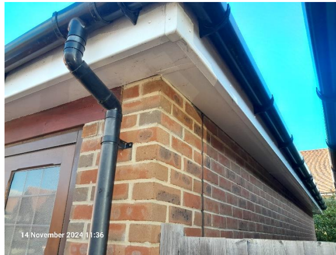
B2: well sealed soffits and brickwork intact, southern elevation (left).
