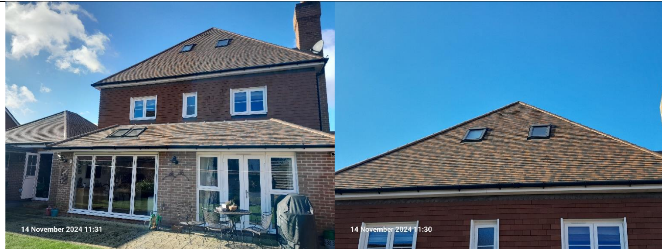
B1: Eastern elevation (left) and up close of flat roof tiles representative of the whole roof (right).
