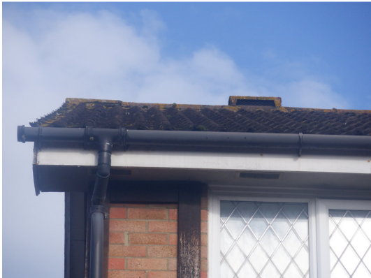
Photograph 5. Vented ridge tile covered by a wire mesh (front elevation).
