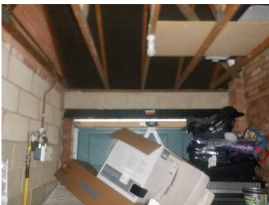
Photograph 20. Open eaves along front elevation (garage).
