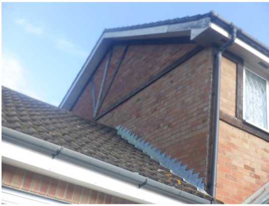
Photograph 7. Lead flashing sealed along garage (western elevation).
