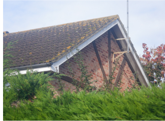
Photograph 4. Fully sealed interlocking tiles and intact ridge and verge mortar (eastern elevation).
