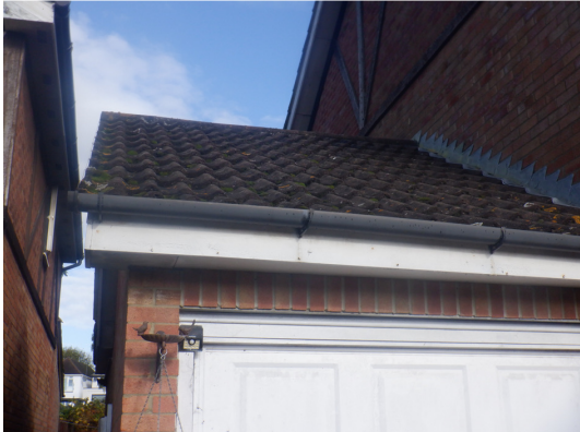
Photograph 3. Fully sealed interlocking tiles (front elevation).
