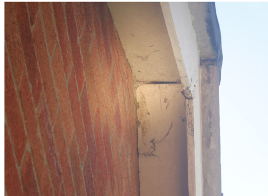
Photograph 11. Gap at apex of gable filled with mortar (west elevation).
