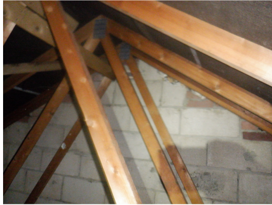
Photograph 12. Roof void of trussed construction.
