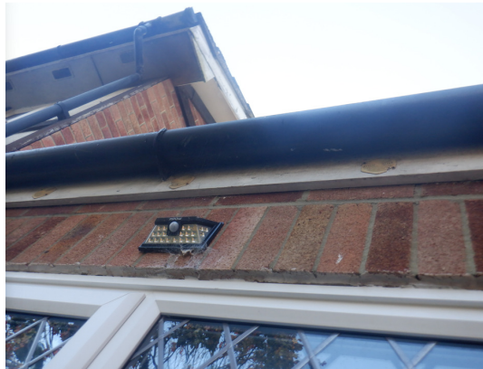
Photograph 9. Timber fascia sealed along the rear flat roof extension (rear elevation).
