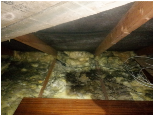
Photograph 15. Eaves filled with fibreglass insulation.
