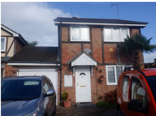
Photograph 1. Front elevation of the house, viewed from the south.
