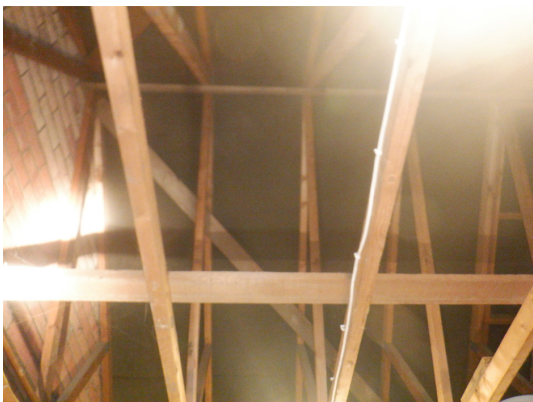
Photograph 18. Open roof garage of trussed construction.
