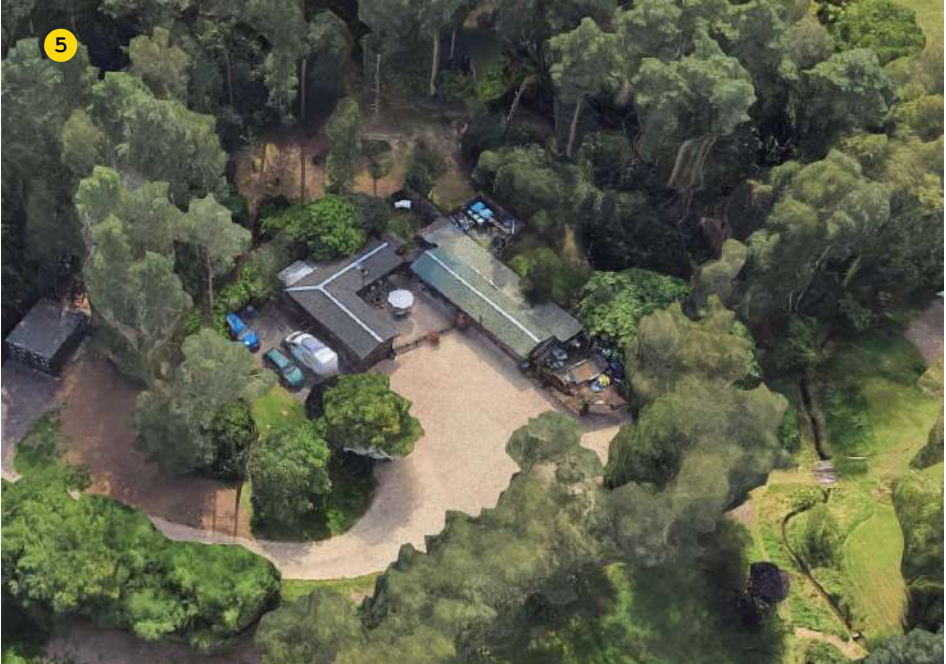
The existing structures on the site comprise two residential units, converted from existing stables which make a limited positive contribution to the character of the area.
