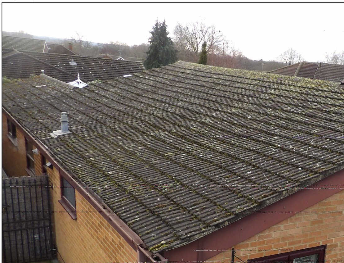
Figure 4. Example of sealed roof and ridge tiles. 79 Wessex Gardens, Twyford. 14.01.25
