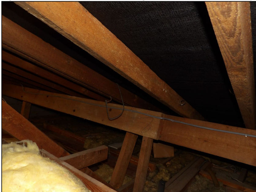
Figure 10. Example of bitumen lining. 79 Wessex Gardens, Twyford. 14.01.25
