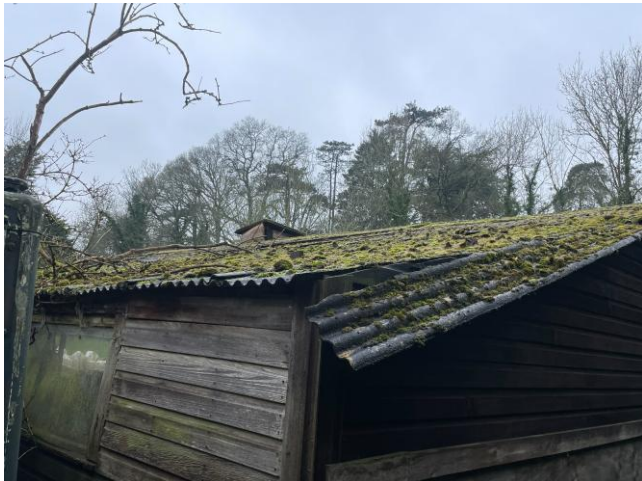
Photo 12c: Showing the roof of B1 with no missing tiles or tile gaps.
