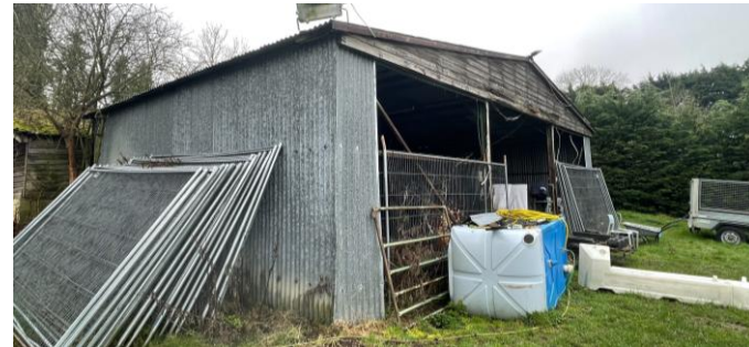
Photo 12a. Showing the exterior of B2.
