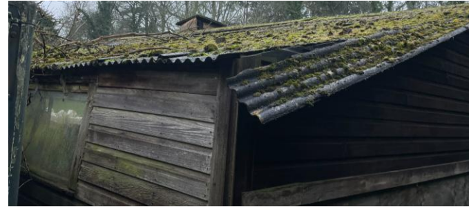
Photo 11c. Showing the roof of B1 with no missing tiles or tile gaps.
