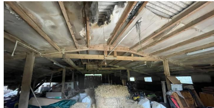
Photo 11d. Showing the interior of B1
