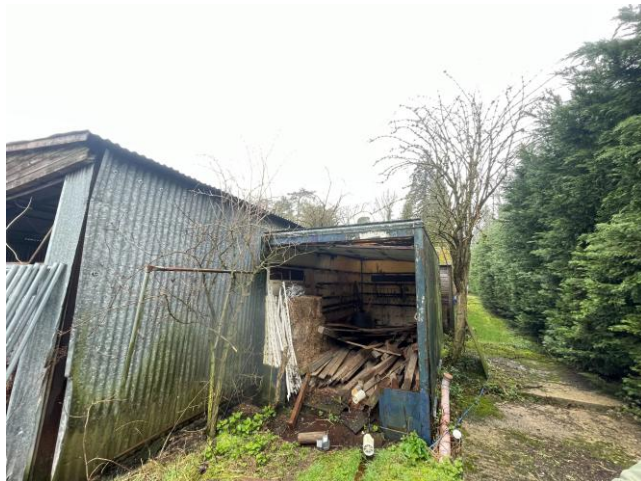
Photo 10: Showing T11 adjacent to the eastern side of B2.
