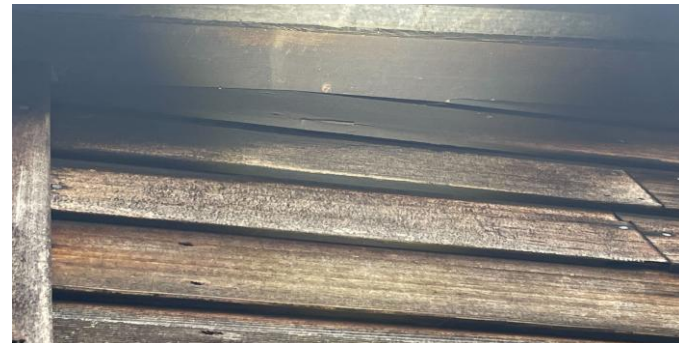
Photo 11b. Showing the woodend cladding of the building with no gaps present.
