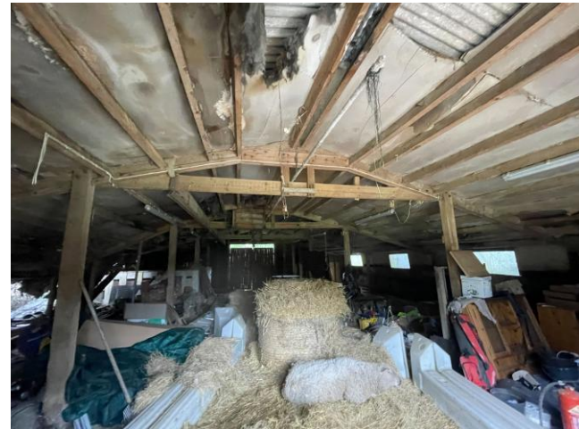
Photo 12d: Showing the Interior of B1.
