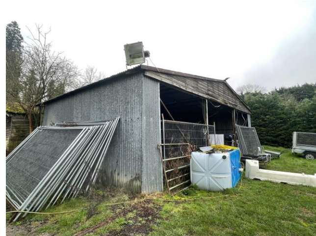
Photo 12a. Showing the exterior of B2.
