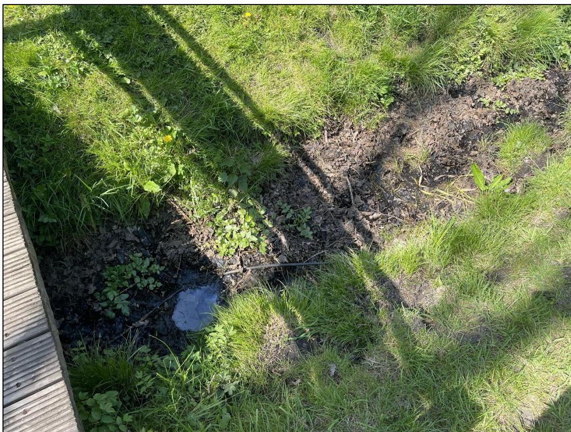
Plate 3 – Dry ditch along northern and western site boundary
