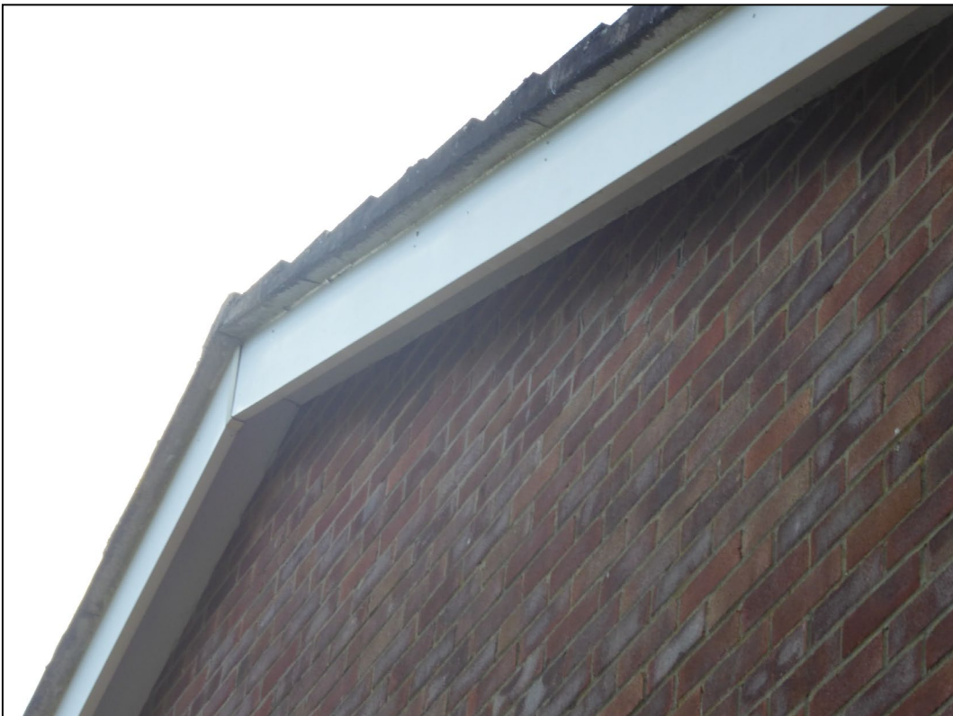
Figure 7. Sealed soffits/fascias. Lancambria, Basingstoke Road, Swallowfield. 05.08.24
