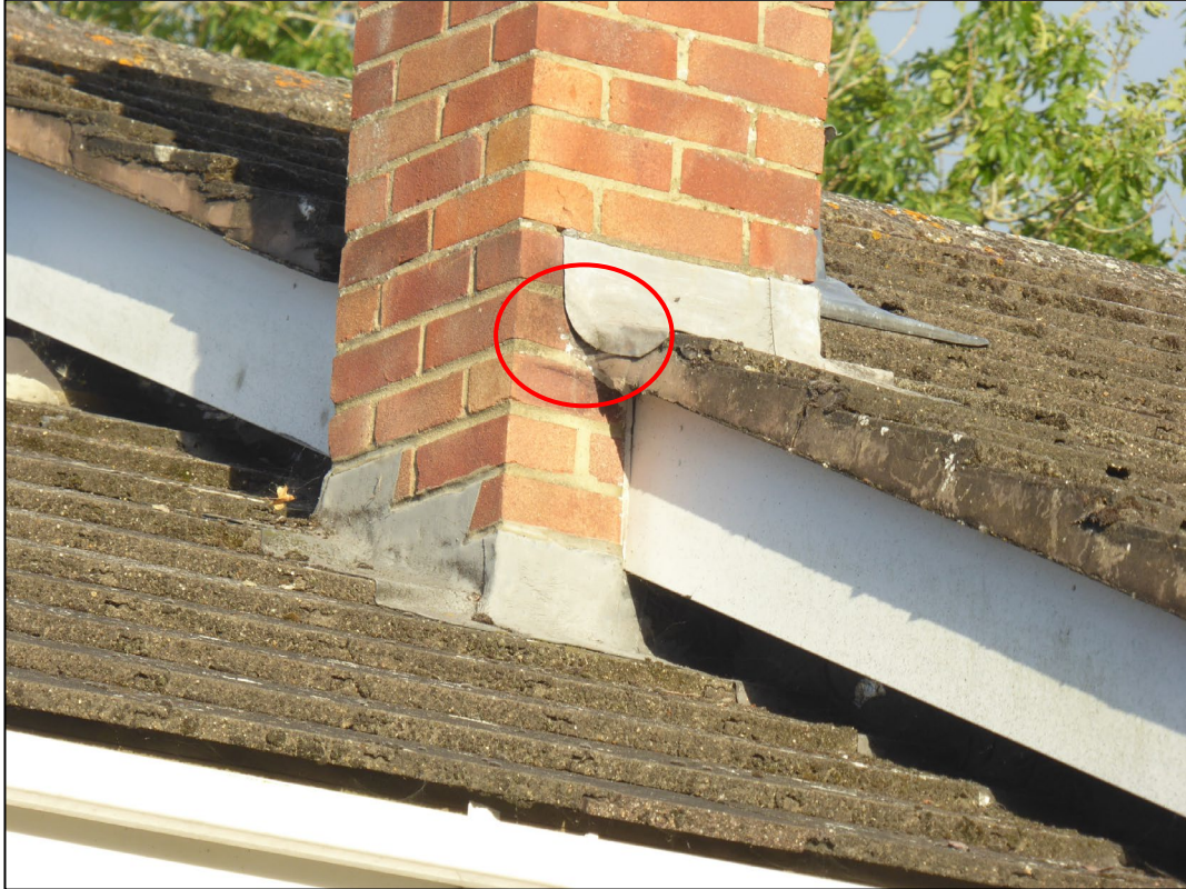
Figure 6. Raised lead flashing on rear chimney stack. Lancambria, Basingstoke Road, Swallowfield. 05.08.24
