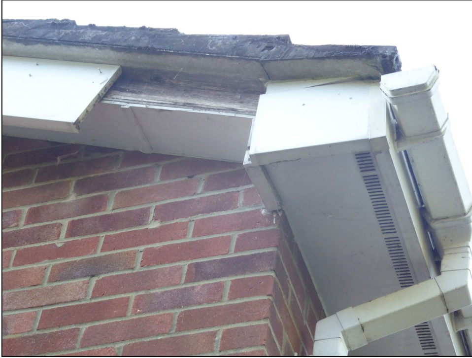
Figure 8. Missing fascia on southern gable end. Lancambria, Basingstoke Road, Swallowfield. 05.08.24
