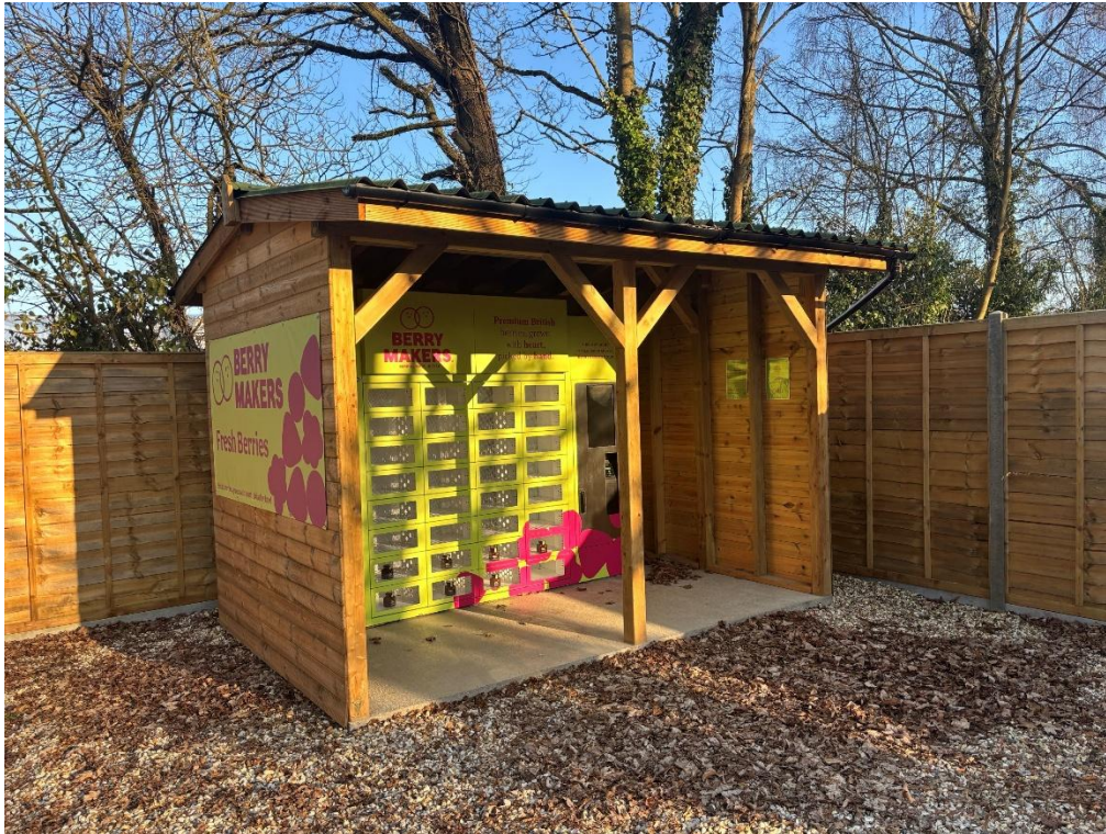
Photo.5 – Vending machine structure
