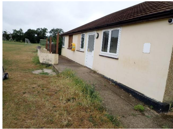
4. The pavilion building and associated hard standing.
