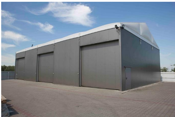
Typical external view
