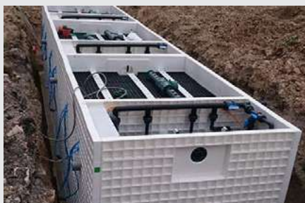
► Treatment plant during installation.
