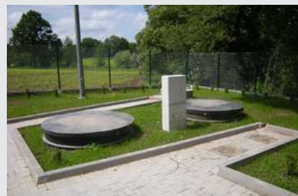
► Remote settlement and buffer tanks to suit a site with restricted space.
