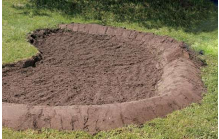
A berm built around the downhill sides of a rain garden helps hold stormwater. The rain garden soils have been amended with sand and a planting soil mix.
