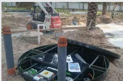
► Treatment plant during installation.
