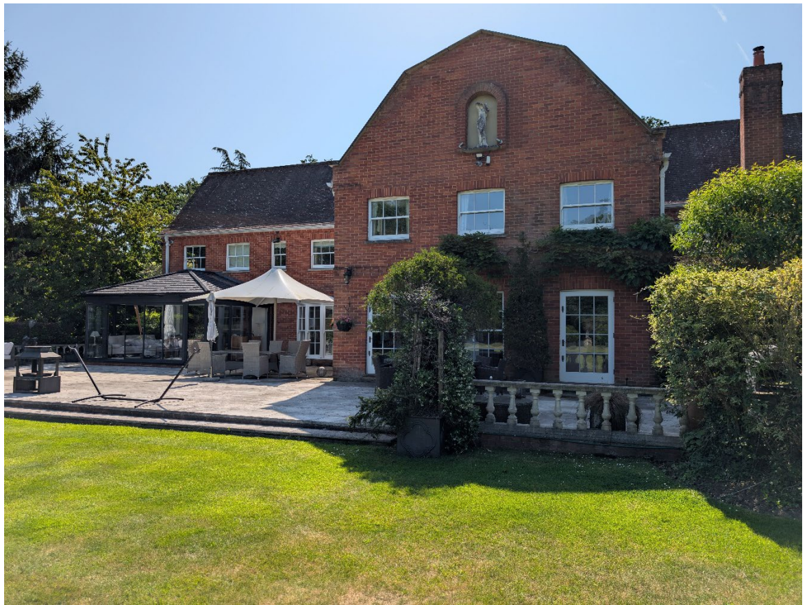
Existing Rear View from West with solid roofed conservatory
