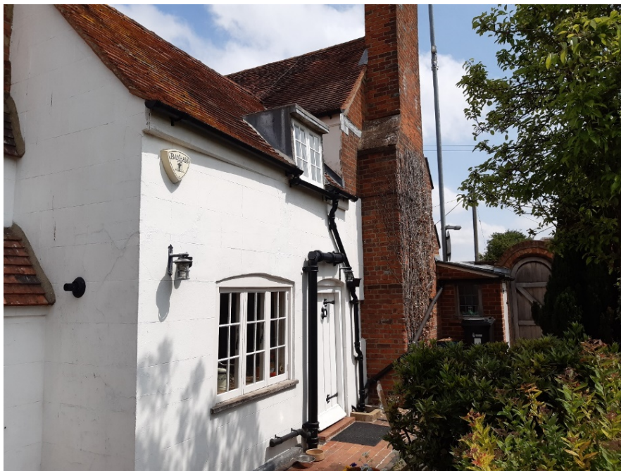
Figure 2 South side elevation of Highway Cottage
