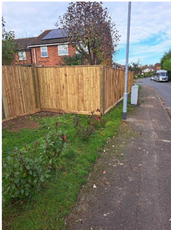
Figure 1.0 – Case Officer site visit photo dated 14 th November 2024 showing the unauthorised development.
