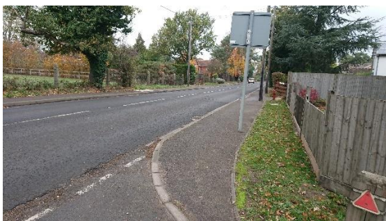
Photograph 2: Looking north on Reading Road
