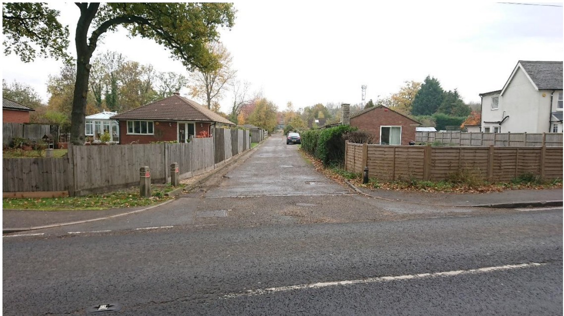
Photograph 1: Existing Site Access
