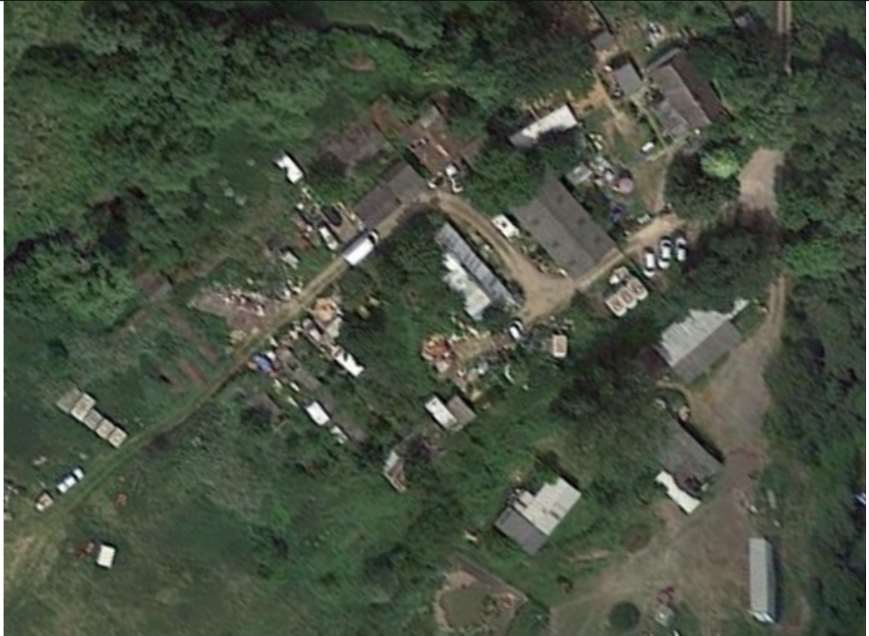
Figure 7 – 2018 Aerial - All structures and caravans visibly in situ. Caravan 2 is not visible. The 3no. structures (labelled as 1 shaded in red) are in a different position.
