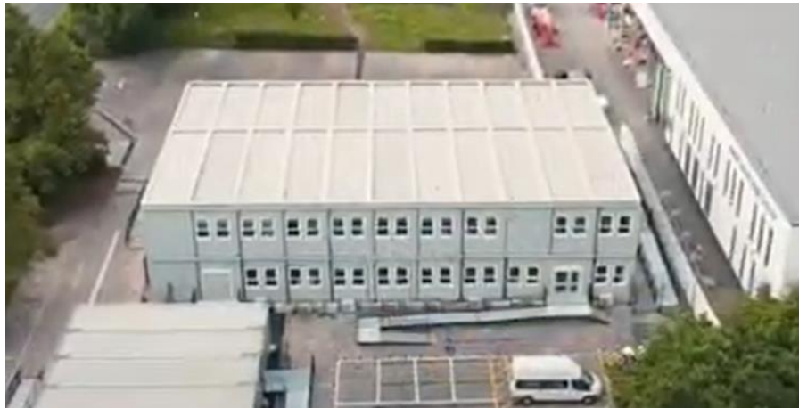
Example of modular or double stacked office arrangement
