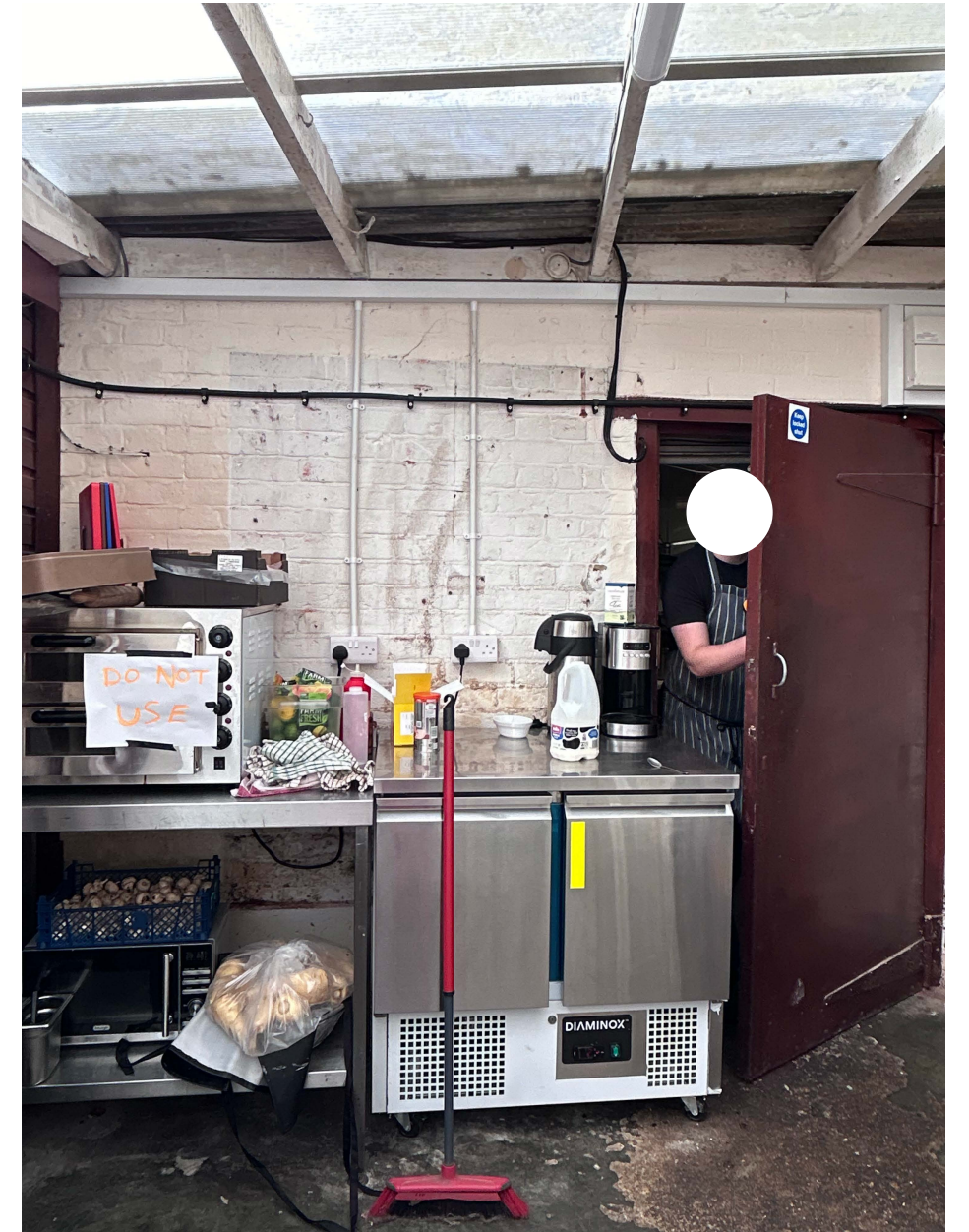
Fig. 41, Kitchen Store, as existing.
