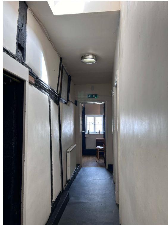
Fig. 34, Corridor, original east elevation seen to right.
