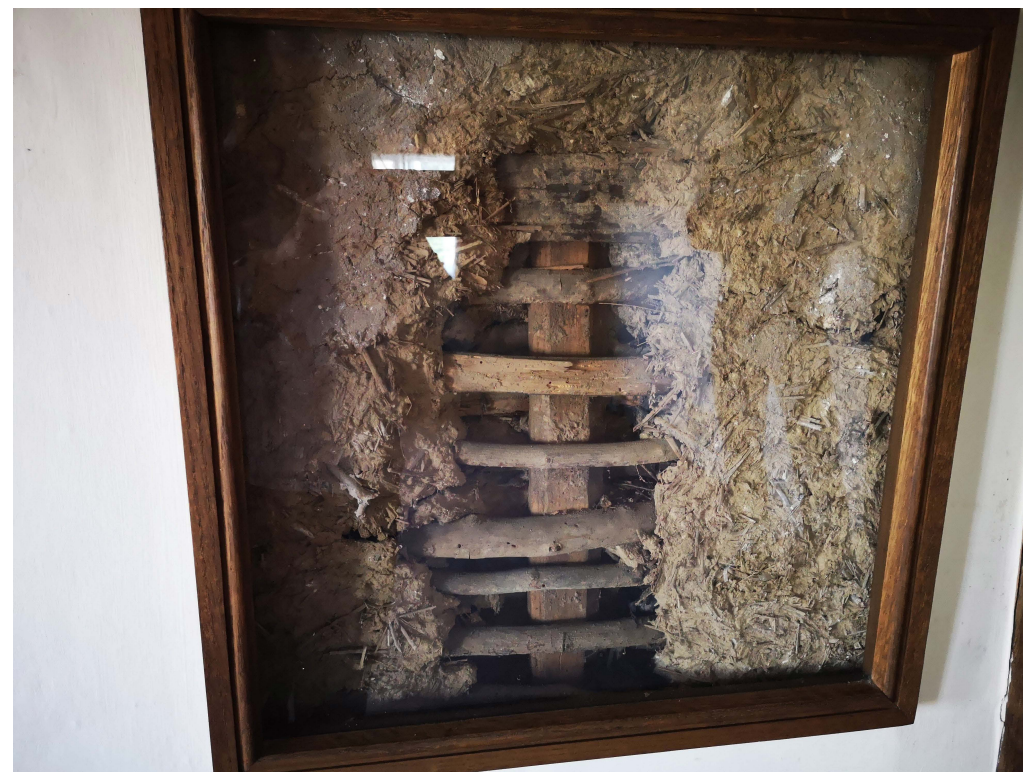
Fig. 43, Wattle and daub framed feature.
