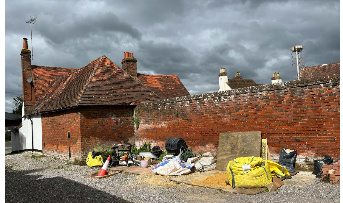
Fig. 25, Extension at the rear, as seen from south. Garden wall adjoining the early 19th century extension.
