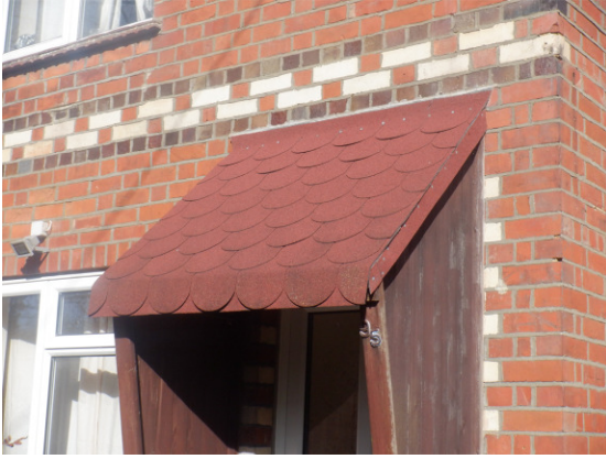
Photograph 5. Porch covered by a flat felt (front elevation).
