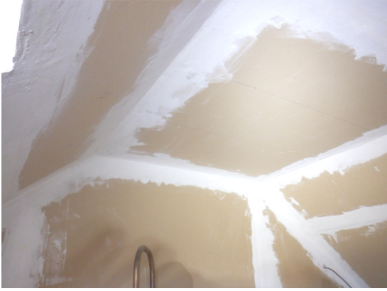
Photograph 11. Central roof void with plasterboard lining.
