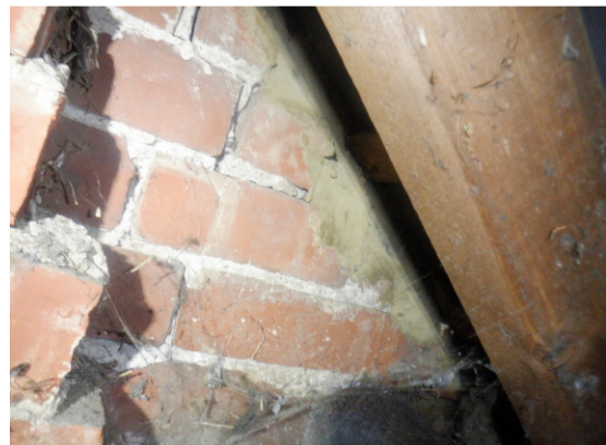
Photograph 15. Edges of the brickwork gables sealed by mortar (northeast eave space).
