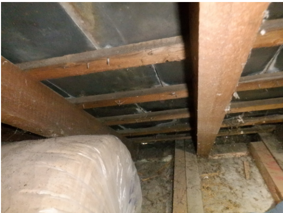
Photograph 13. Daylight within the eaves (southwest eaves space).
