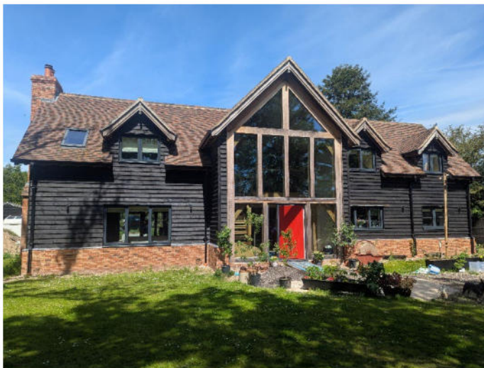
Figure 3: Replacement dwelling almost completed
