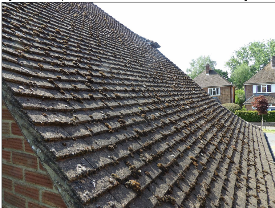
Figure 4. Example sealed roof tiles. 26 Priest Avenue, Wokingham. 13.05.25
