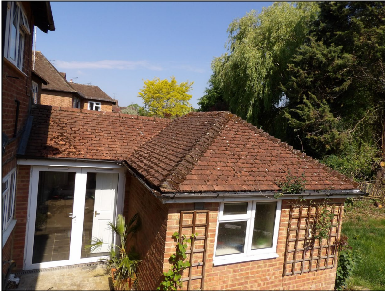
Figure 10. Example sealed roof tiles on rear extension. 26 Priest Avenue, Wokingham. 13.05.25
