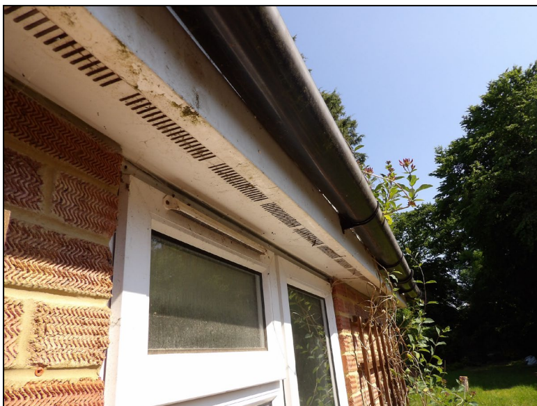
Figure 11. Example sealed soffits and fascias on rear extension. 26 Priest Avenue, Wokingham. 13.05.25
