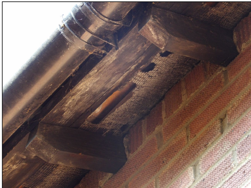
Figure 8. Example rotten bitumen covering eaves. 26 Priest Avenue, Wokingham. 13.05.25
