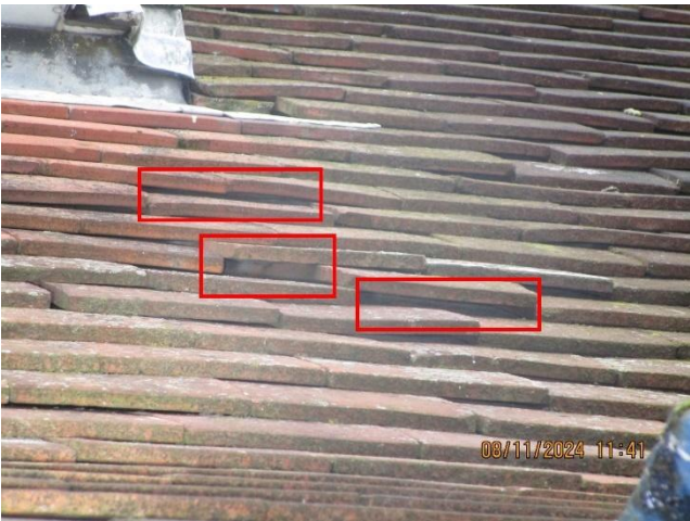
Photos 11 and 12 – Example of gaps under roof tiles
