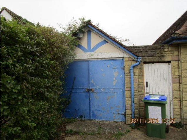
Photos 9 and 10 – Example of missing verge mortar at the front gables of the bungalow
