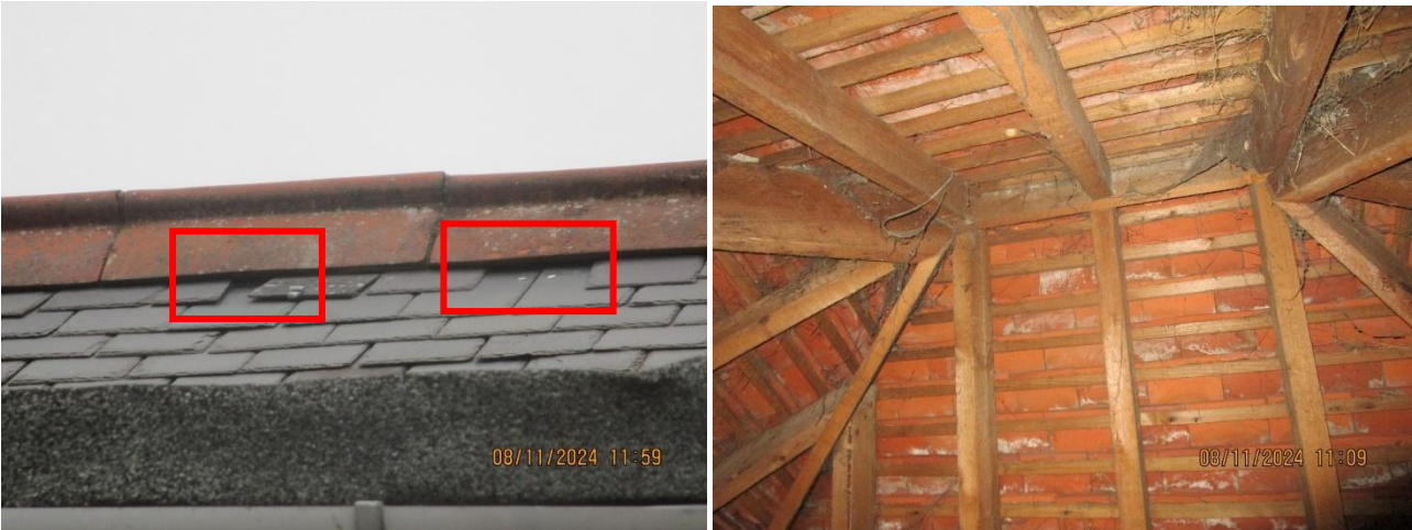
Photos 21 and 22 – Inside the eaves level loft space
