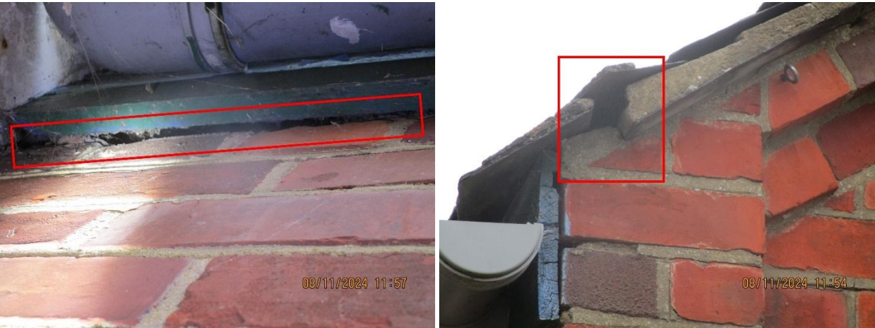
Photo 17 – Gaps under slipped slate tiles on the northeastern elevation of the Church hall, and Photo 18 – Gaps under hip tiles on the northeastern elevation of the Church hall
