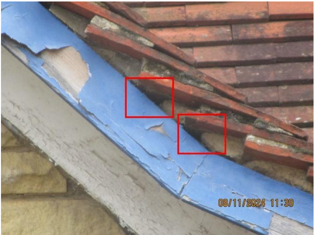
Photos 9 and 10 – Example of missing verge mortar at the front gables of the bungalow
