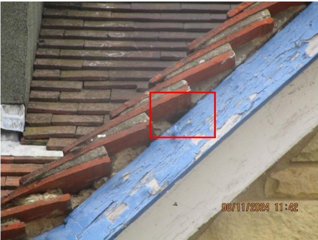
Photos 11 and 12 – Example of gaps under roof tiles
