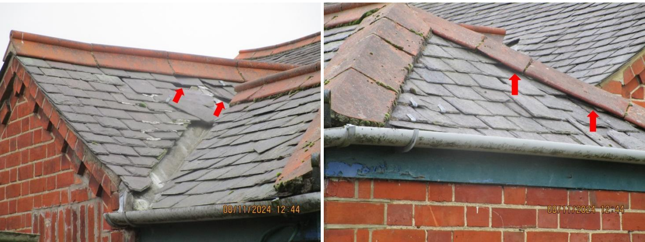
Photo 17 – Gaps under slipped slate tiles on the northeastern elevation of the Church hall, and Photo 18 – Gaps under hip tiles on the northeastern elevation of the Church hall
