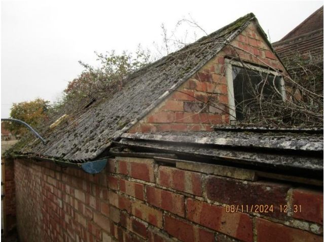
Photos 9 and 10 – Example of missing verge mortar at the front gables of the bungalow
