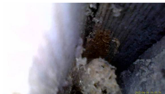
Photograph 2. Endoscope behind barge board.
