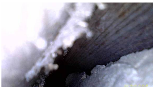
Photograph 1. Endoscope behind barge board.
