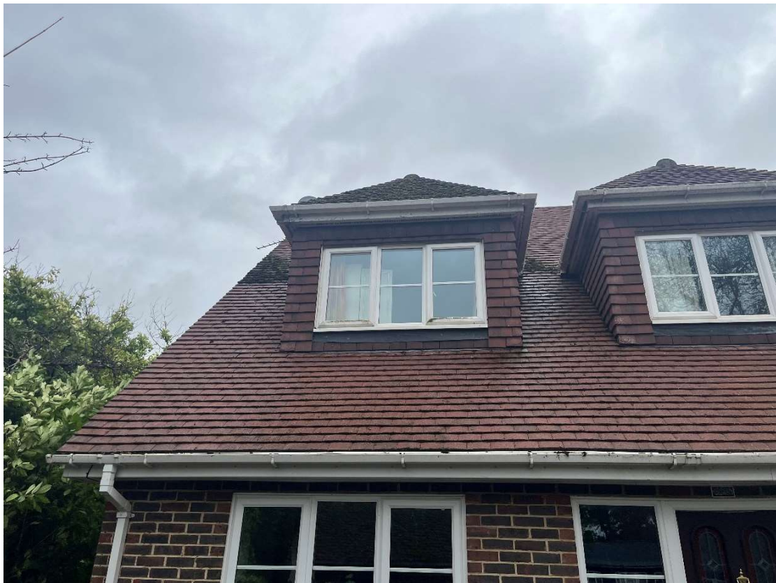
Figure 4. Northern elevations (eastern half) looking south.
