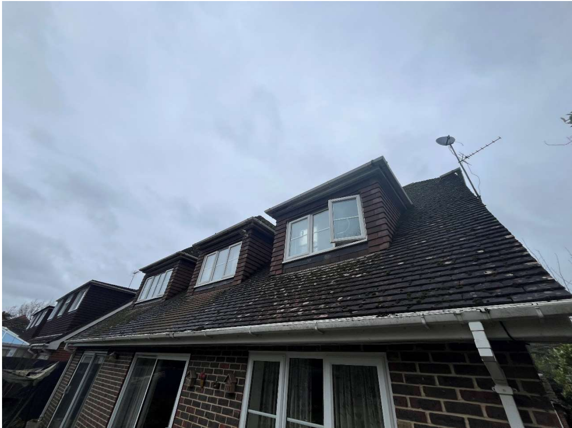
Figure 3. Southern and eastern elevations looking north.
