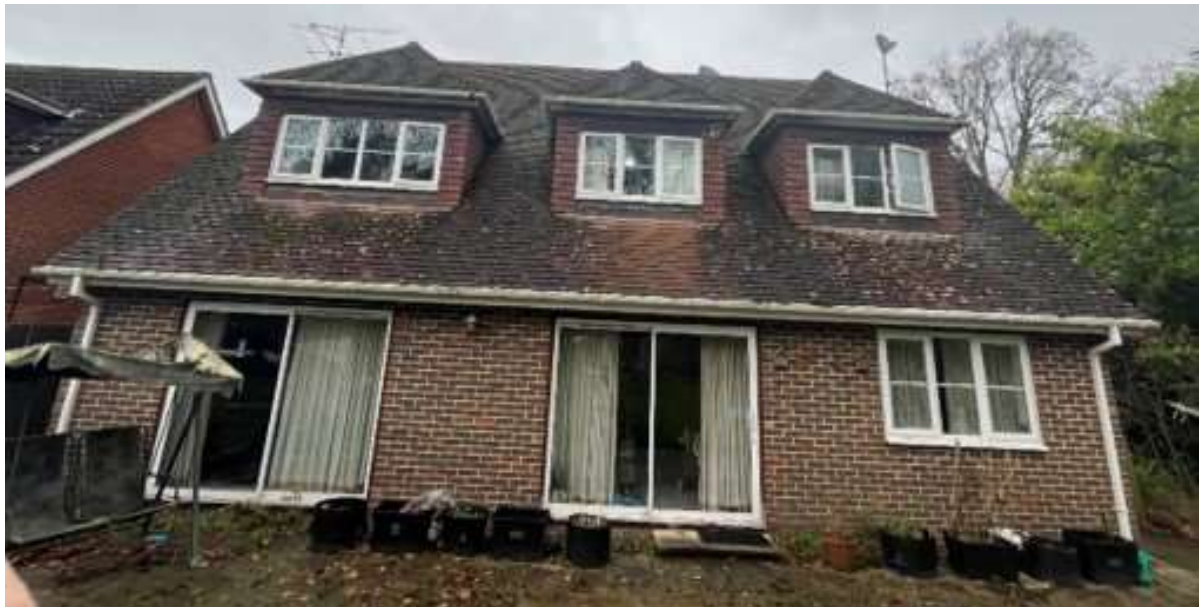
Figure 2. Southern elevations looking north.
