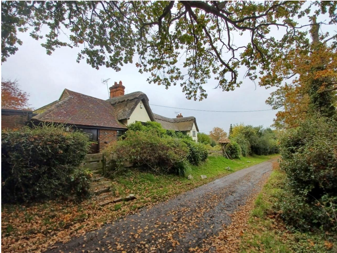
Fig 1 – Existing dwelling from Drift Lane.
