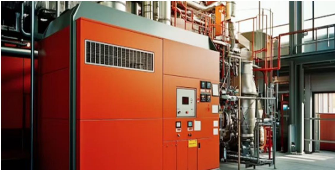
Figure 3.3: Combined Heat and Power (CHP) Plant
