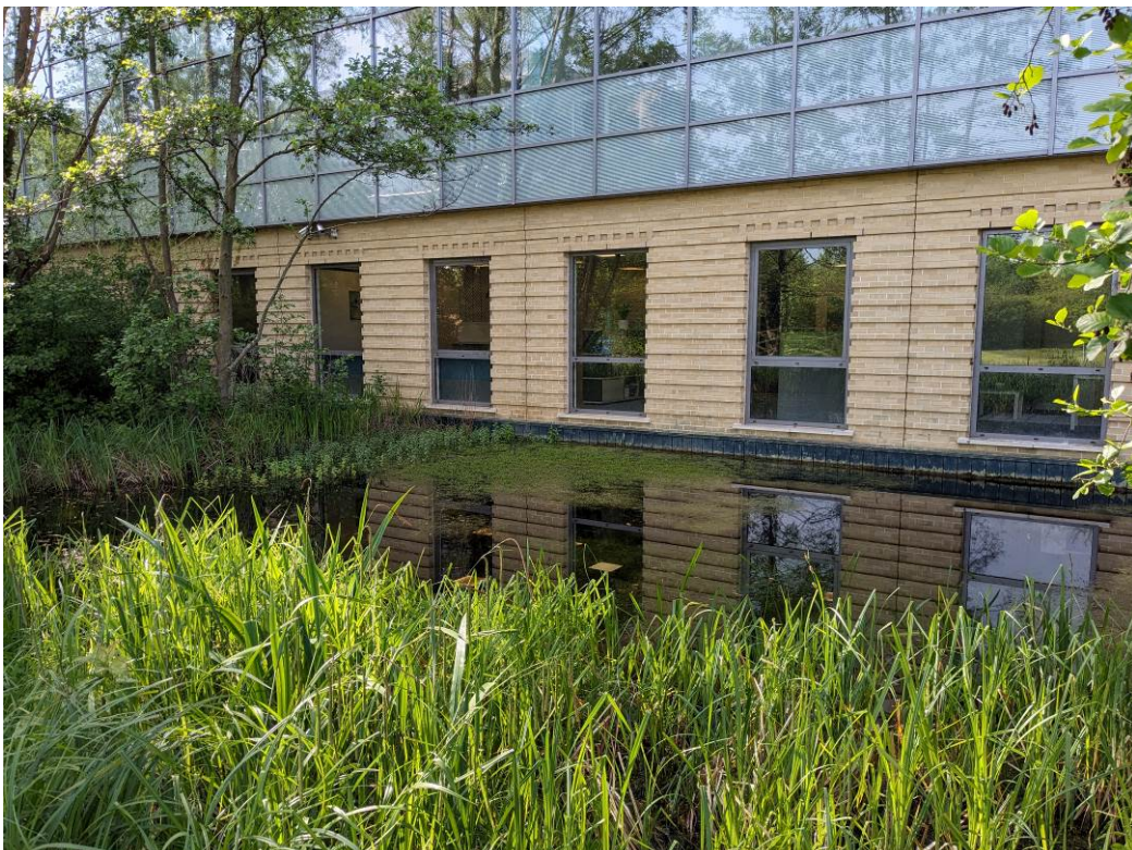
Photograph 2 – Pond within north
