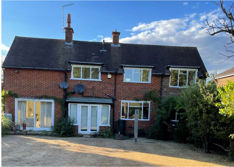
Photograph showing the rear elevation.
