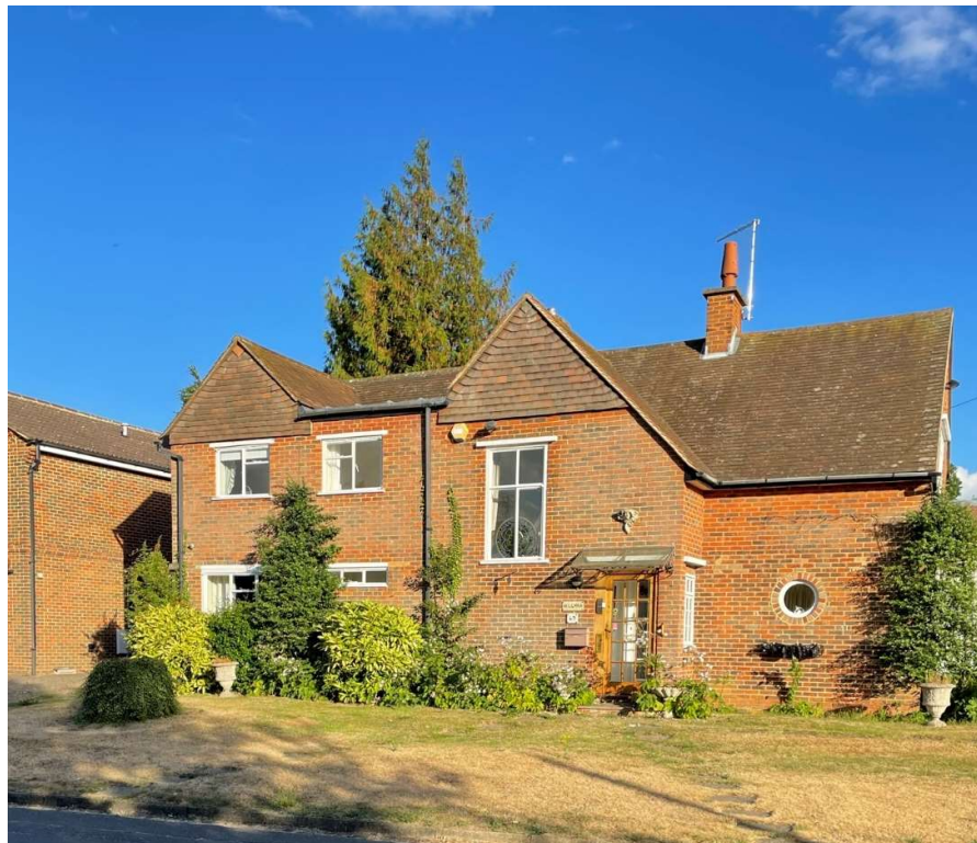
Photograph showing the front elevation.
