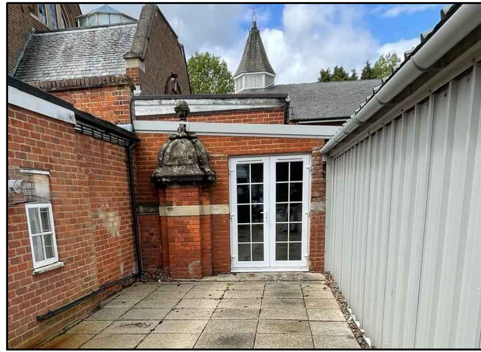
EXTERNAL VIEW OF BRICK PIER
