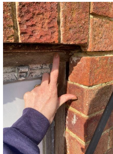
Figure 7: Example of potential roosting feature within building on Site
