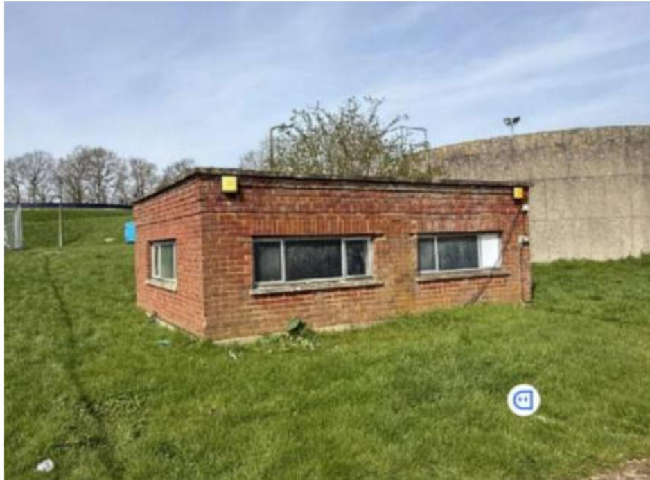
Figure 1 – Photograph of Sludge Pumphouse Building to be demolished
