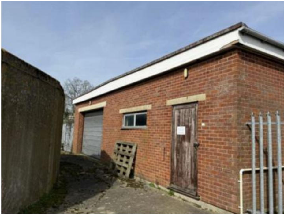
Figure 3 – Photograph of R&D Workshop to be demolished
