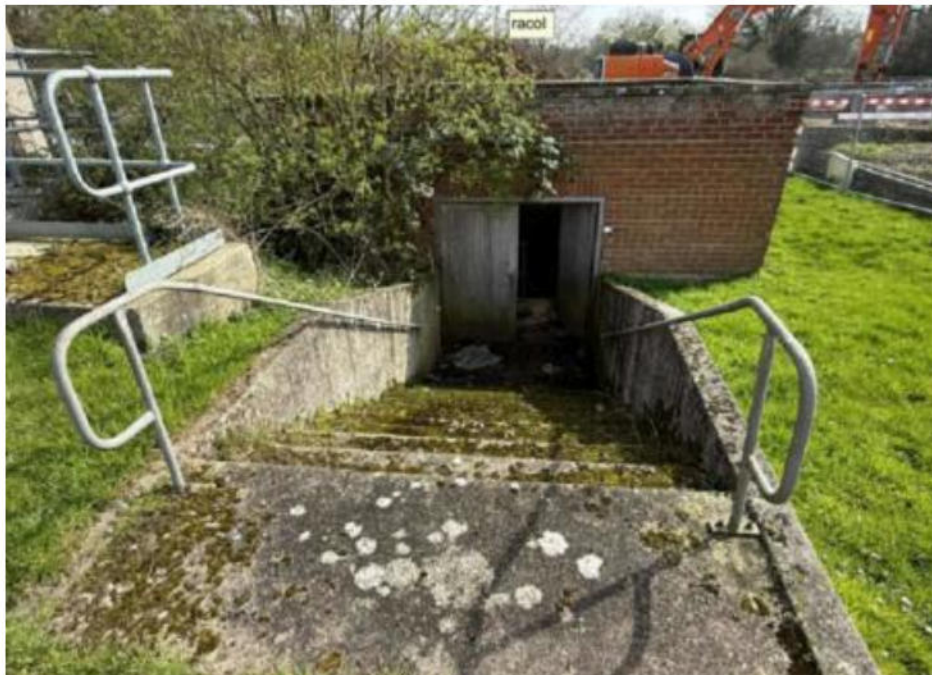
Figure 2 – Photograph of Disused Sludge Pumphouse Building Access
