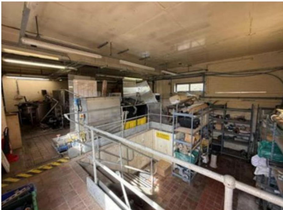
Figure 4 – Internal photograph of R&D Workshop to be demolished
