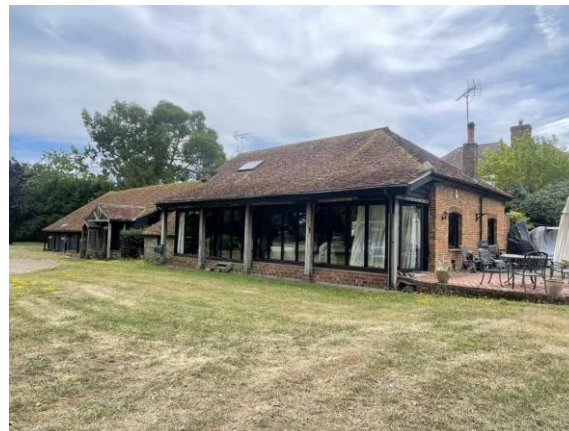
B1- northern and western elevations
