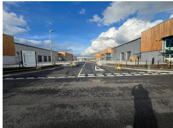
Viscount Way access to main site
