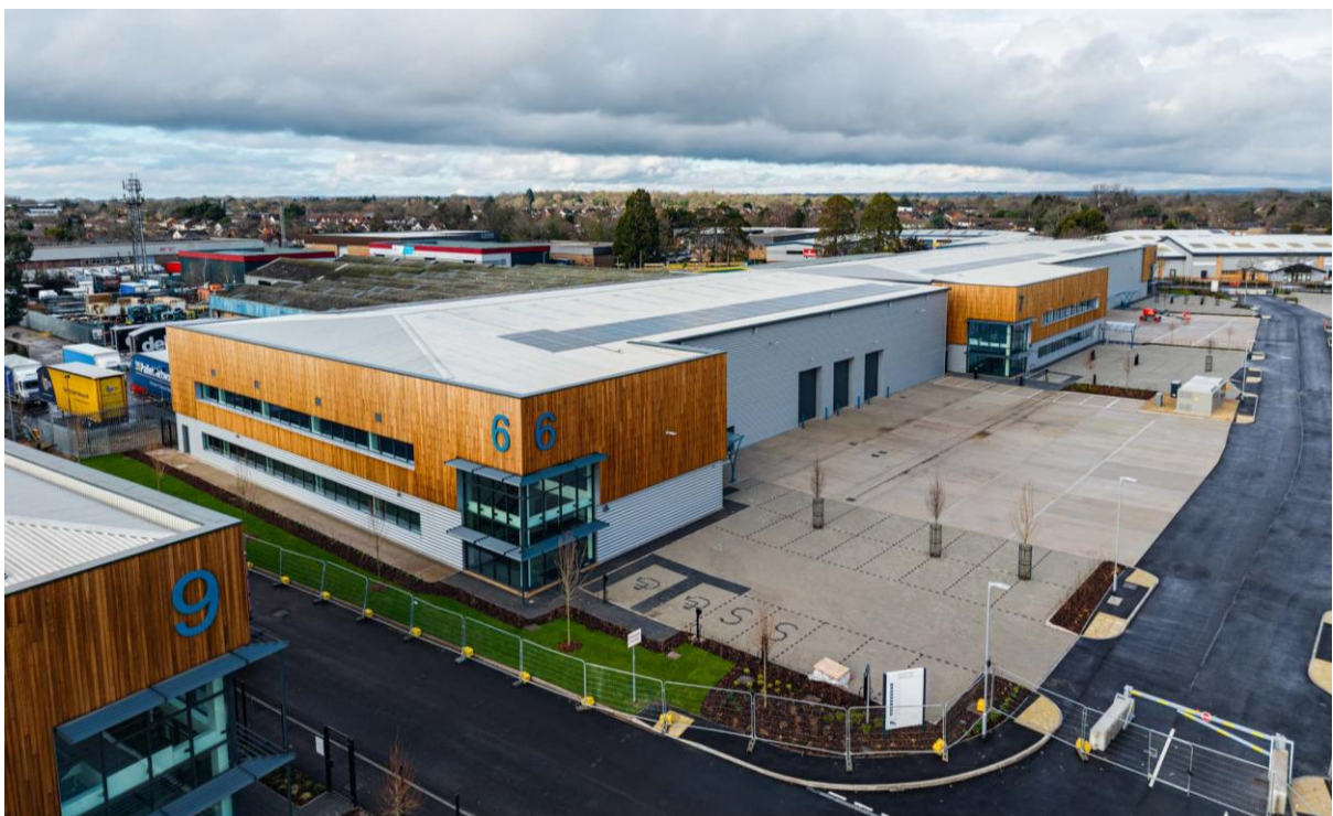
View looking north illustrating complete buildings with cladding shown, windows & curtain walling, block paving, road and yards plus landscaping.
