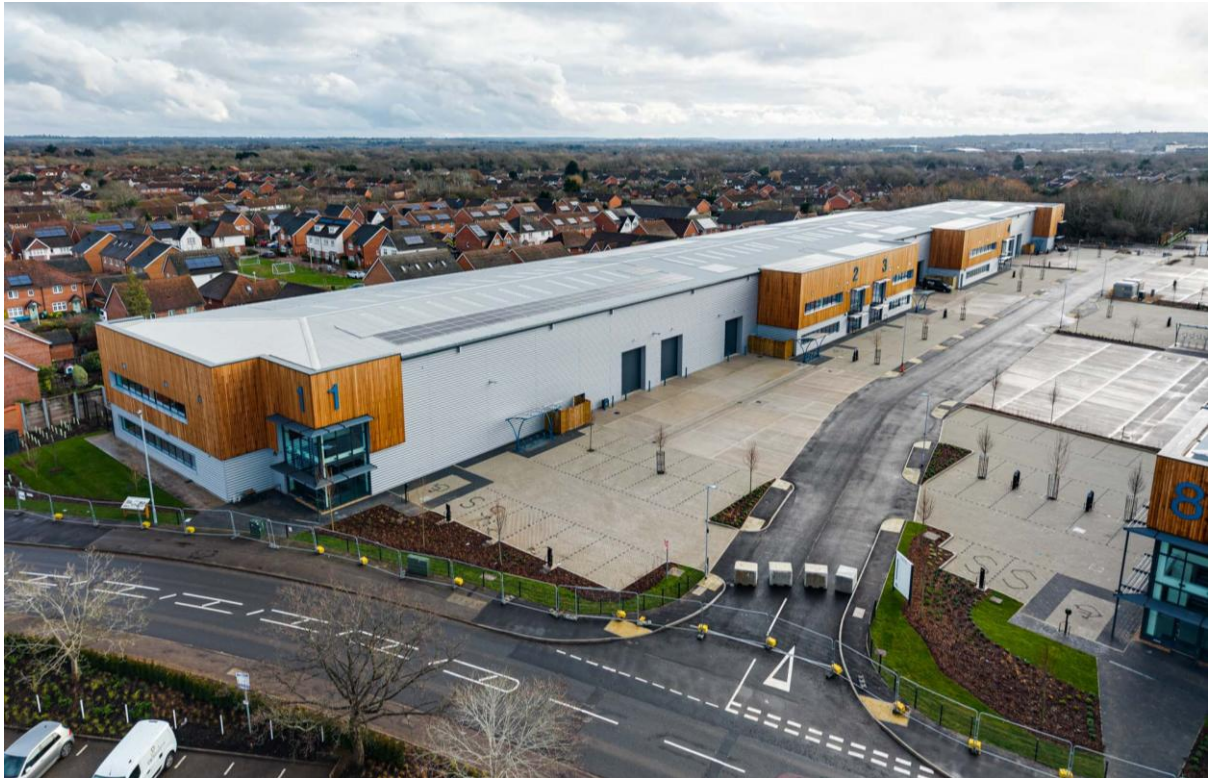
View looking south illustrating complete buildings with cladding shown, windows & curtain walling, block paving, road and yards plus landscaping.
