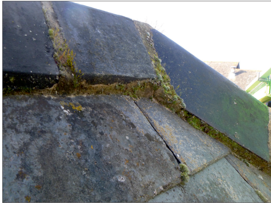
Photograph 2: Showing the close inspection of the ridge and roof tiles, mostly well-sealed, with any restricted gaps found to be filled by moss and general debris.
