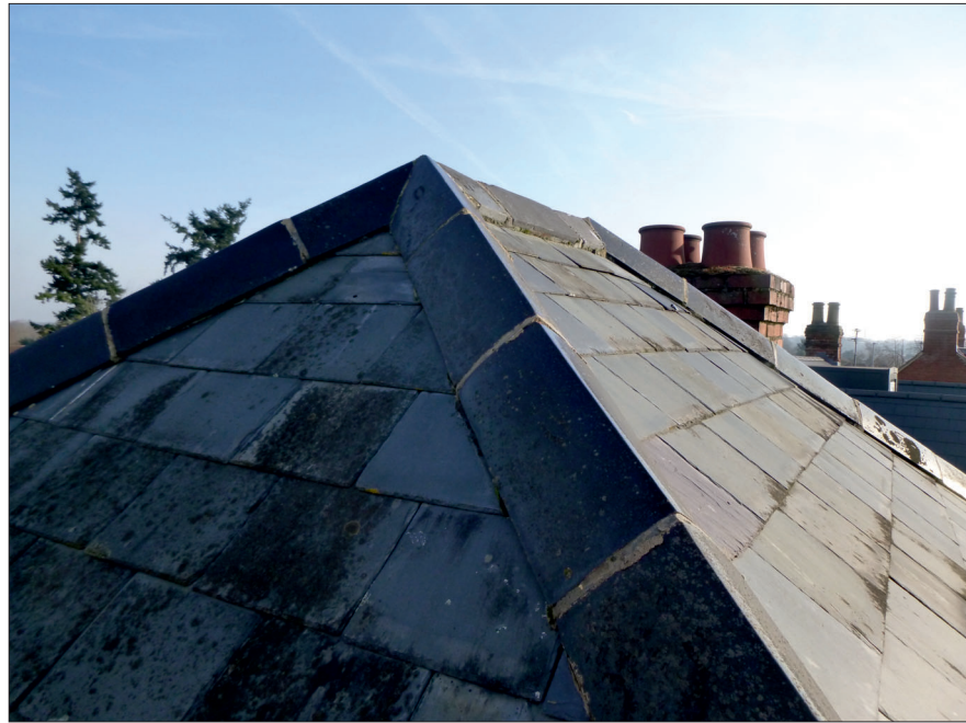
Photograph 1: Showing the close inspection of the roof and ridge tiles on the main residential dwelling, with well-sealed slate tiles.
