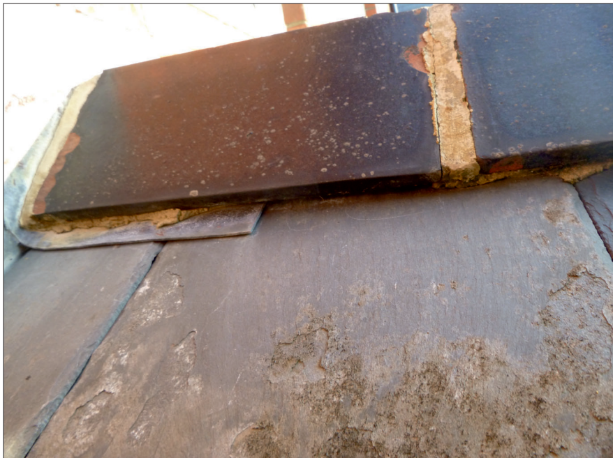
Photograph 8: Showing the well-sealed lead flashing and restricted gap on the single-storey rear extension, thoroughly investigated and found to be shallow and cobwebbed throughout.
