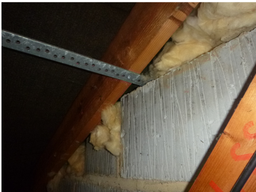
Photograph 12. Gaps around the edges of the blockwork gables filled with fibreglass (roof void).
