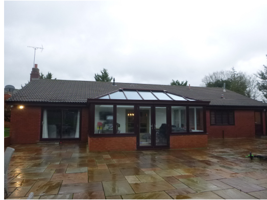
Photograph 2. Rear of property viewed from south.
