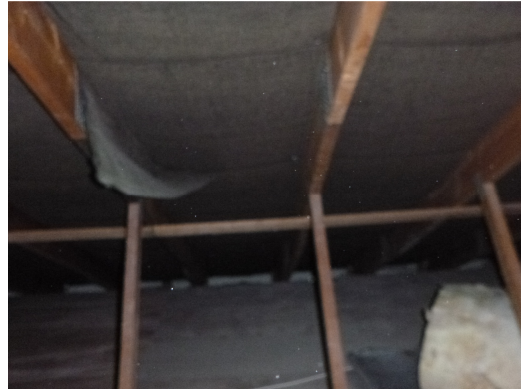
Photograph 9. Roof lining and open soffits (roof void).
