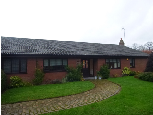
Photograph 1. Front of property viewed from north.
