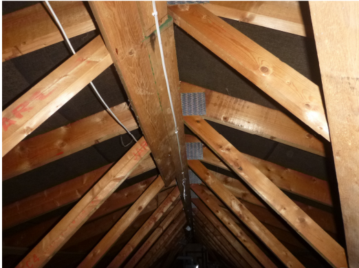
Photograph 8. Roof void of trussed construction.
