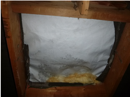
Photograph 10. Removed chimney replaced by a breathable roofing membrane (roof void).
