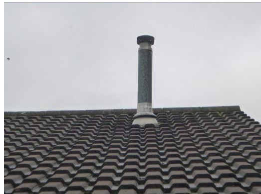
Photograph 4. Slightly raised tiles around flue (rear elevation).
