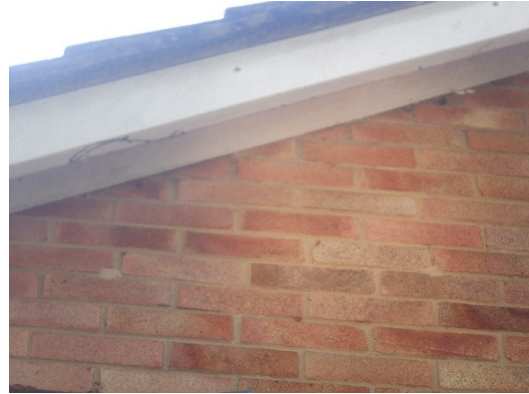
Photograph 6. Tightly fitted soffits (rear elevation).
