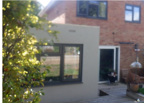
Photograph 12. Rendered extension to the garage (rear elevation).
