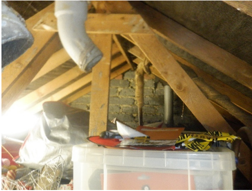
Photograph 15. Roof void showing 'cut and pitch' construction.
