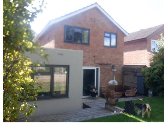
Photograph 2. Rear elevation, viewed from the north.
