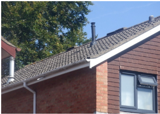
Photograph 3. Tight fitting interlocking concrete tiles with tight ridge and verge (front western elevation)
