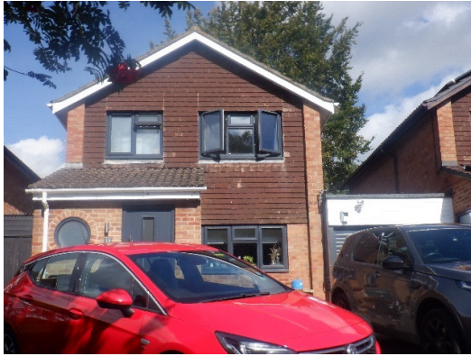
Photograph 1. Front elevation, viewed from the south.
