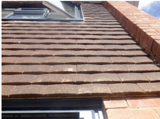
Photograph 7. Tightly fitted flat hanging tiles (front elevation).
