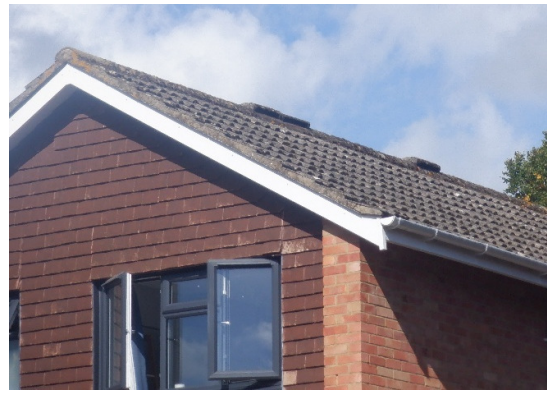
Photograph 4. Ridge and hip mortar fully intact (front eastern elevation).
