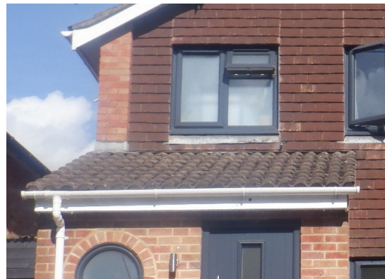
Photograph 14. Flat interlocking porch tiles and top lead flashing (front elevation).
