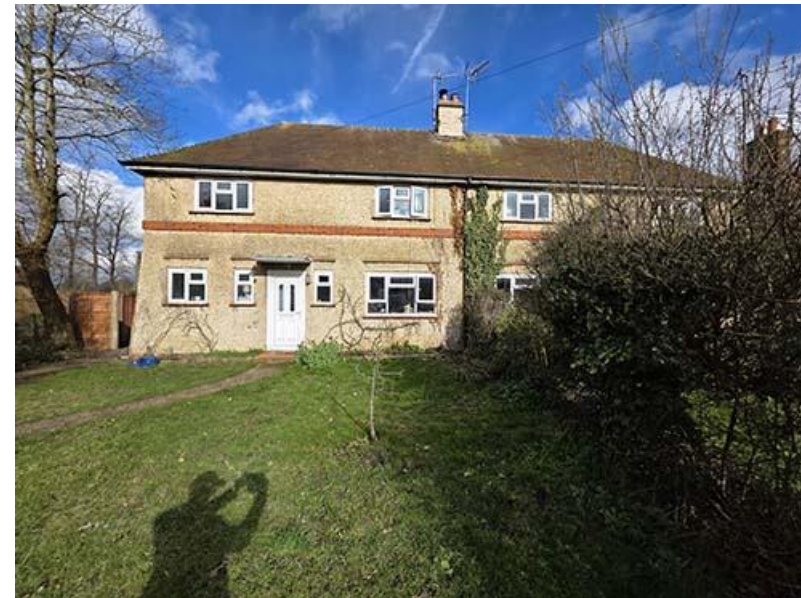
Existing frontage of dwelling
