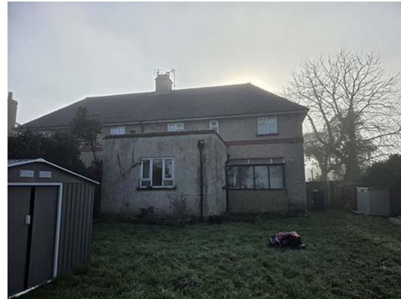
Existing rear extension
