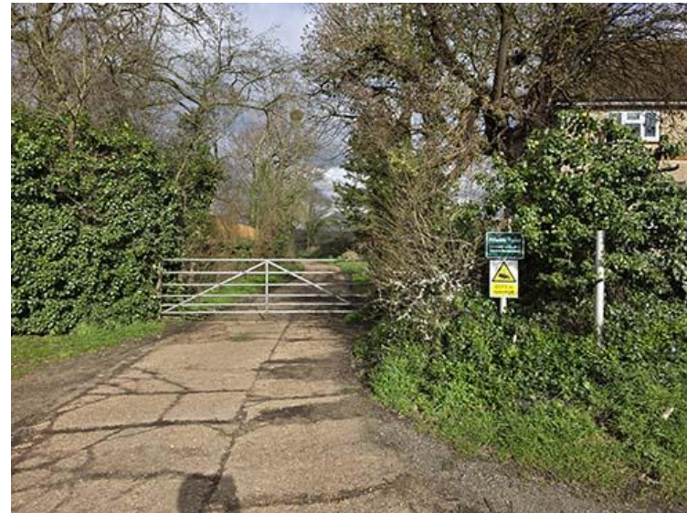
Existing private road – Broadmoor Lane
