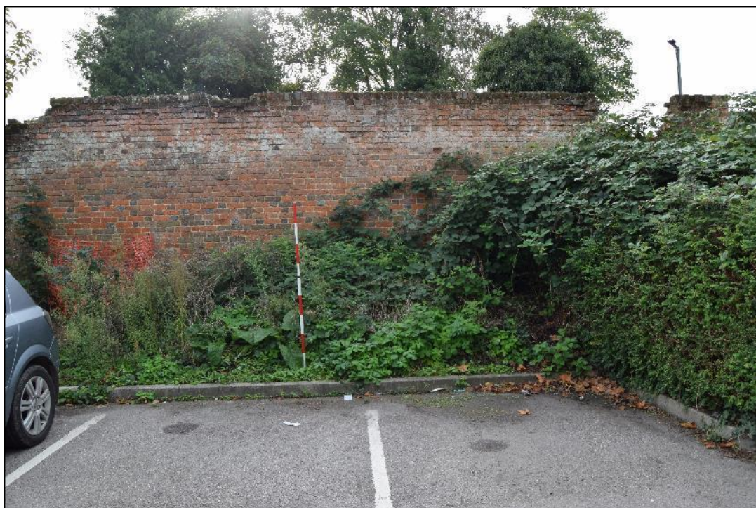
Plate 16: View looking SE towards the NW facing elevation of the wall.
