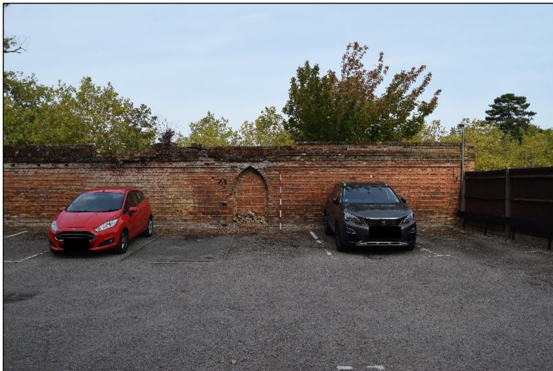
Plate 28: Wide view looking NW towards the SE facing elevation of the wall.
