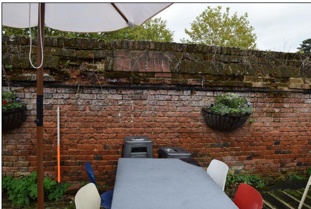
Plate 44: View looking NW towards the SE facing elevation of the wall.
