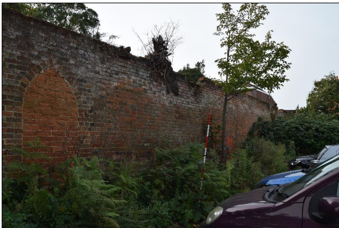
Plate 20: View looking SW along the NW facing elevation of the wall.
