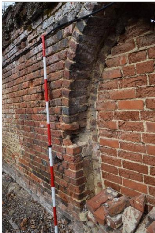
Plate 32: View looking SW towards the SE facing elevation of the wall, focusing on the left side of the infilled archway.
