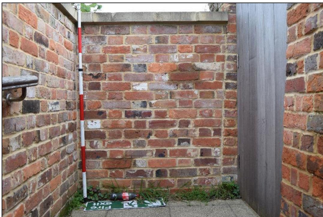
Plate 15: View looking E towards the fire escape to the NW facing elevation of the wall.
