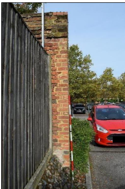
Plate 27: View looking NW towards the SE elevation of the wall.
