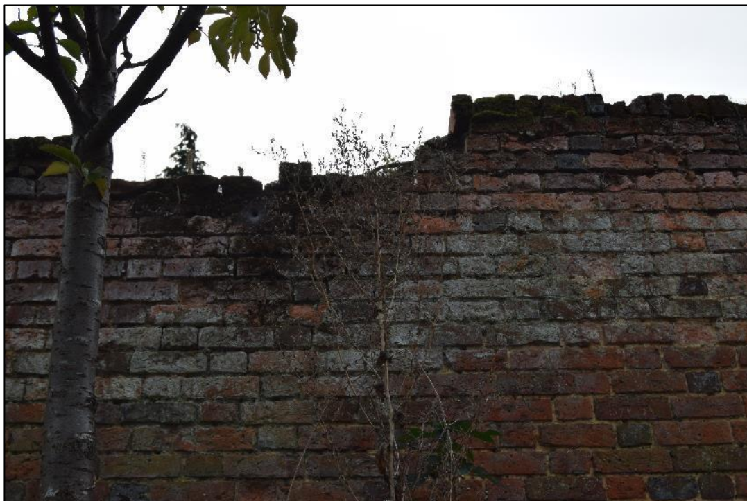
Plate 18: View looking SE towards the NW facing elevation of the wall.
