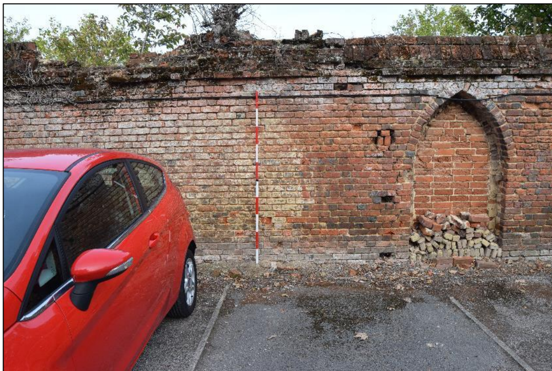
Plate 33: View looking SW towards the SE facing elevation of the wall.
