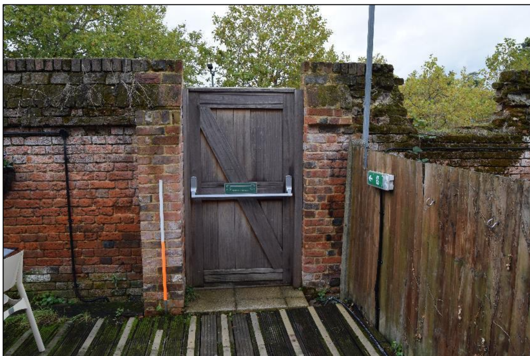
Plate 39: View looking NW towards the SE facing elevation of the wall.
