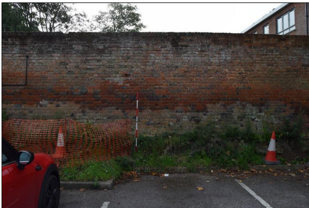
Plate 9: View looking SE towards the NW facing elevation of the wall.
