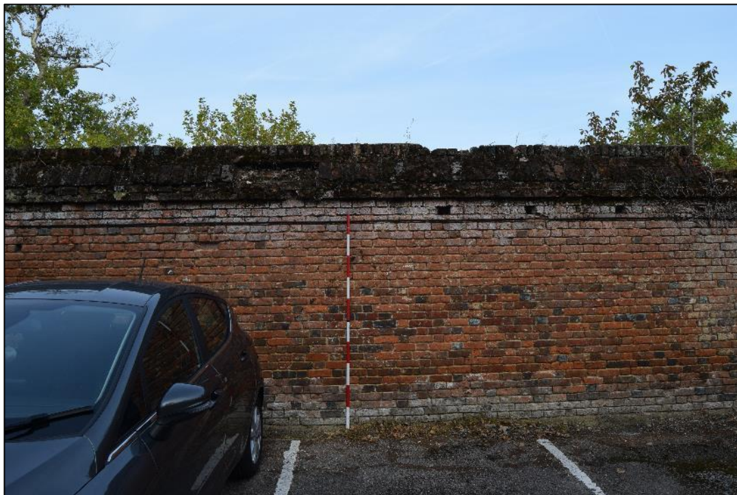
Plate 36: View looking NW towards the SE facing elevation of the wall.
