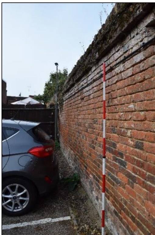
Plate 37: View looking SW towards the SE facing elevation of the wall.
