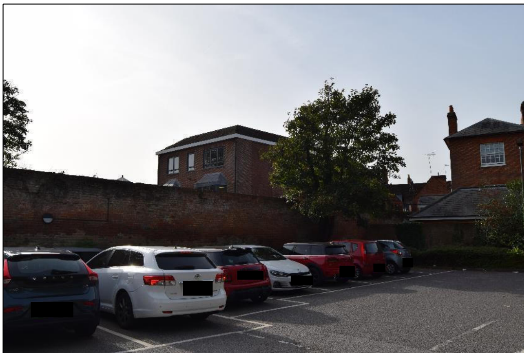
Plate 1: General view of the wall looking SW, with Montague House in the right of frame.
