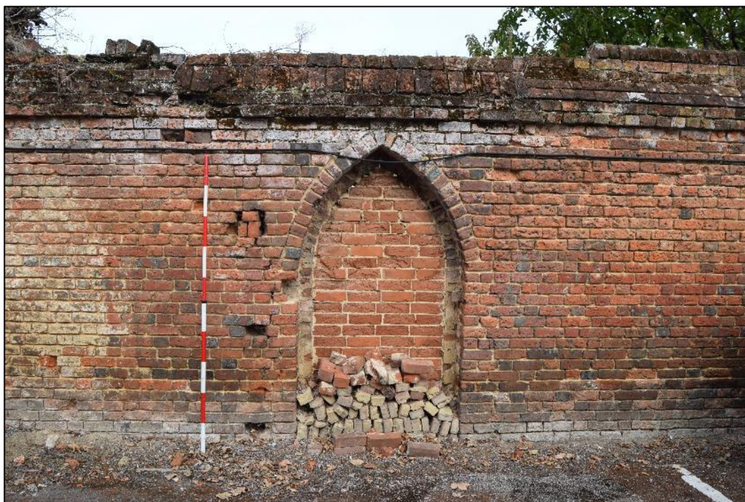
Plate 30: View looking NW towards the SE facing elevation of the wall.
