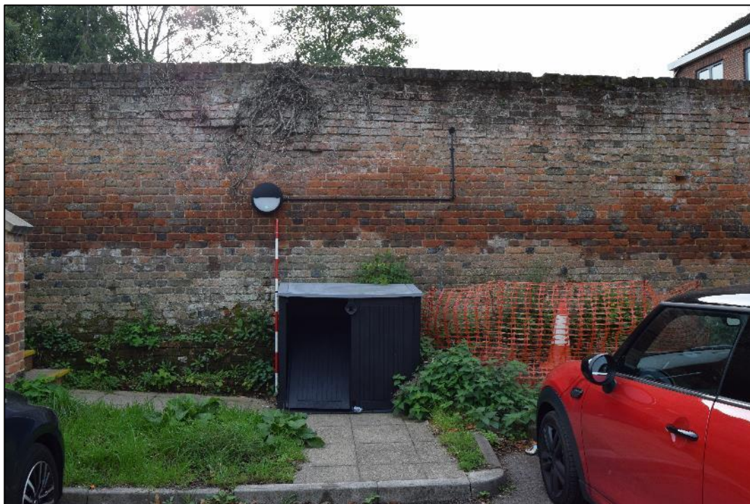
Plate 11: View looking SE towards the NW facing elevation of the wall.
