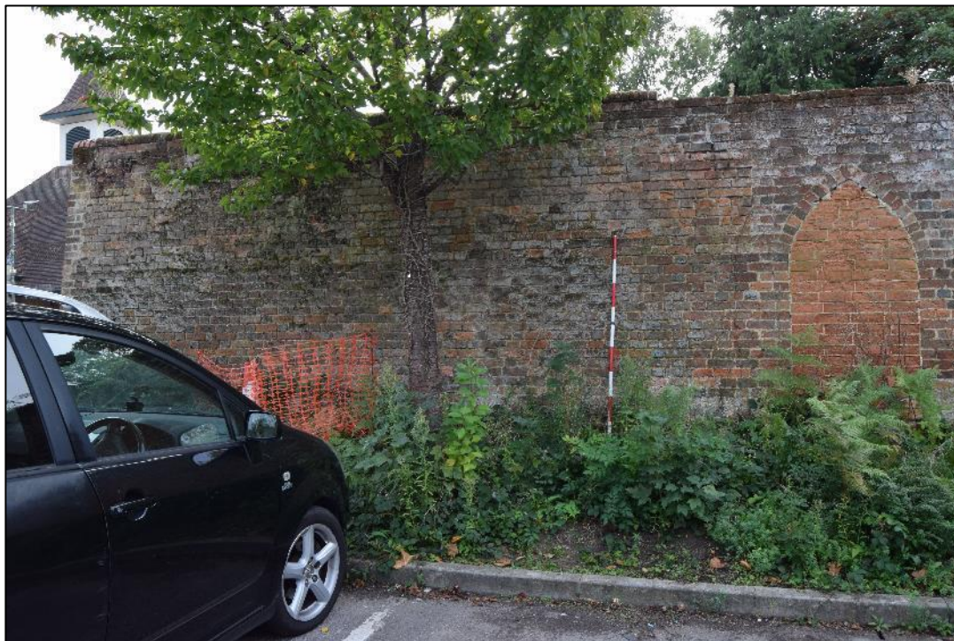
Plate 23: View looking SE towards the NW elevation of the wall.
