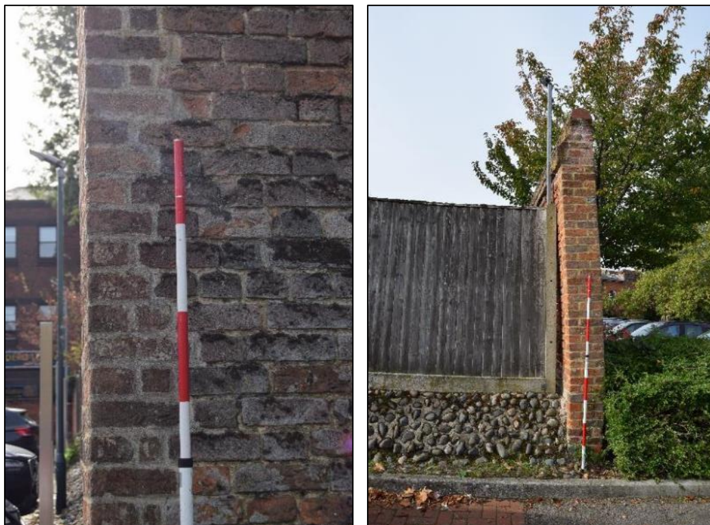
Plate 25 (left): View looking SE towards the NW facing elevation of the wall.
