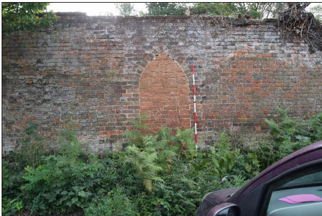
Plate 21: View looking SE towards the NW facing elevation of the wall.
