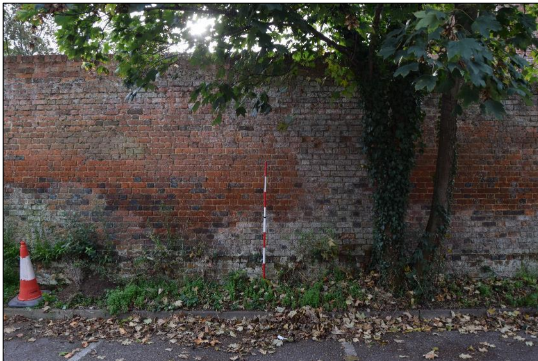
Plate 8: View looking SE towards the NW facing elevation of the wall.
