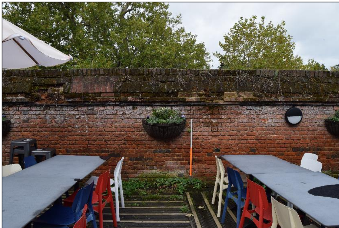
Plate 42: View looking NW towards the SE facing elevation of the wall.
