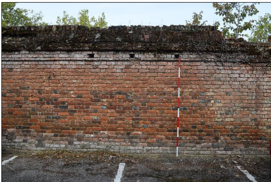
Plate 35: View looking NW towards the SE facing elevation of the wall.
