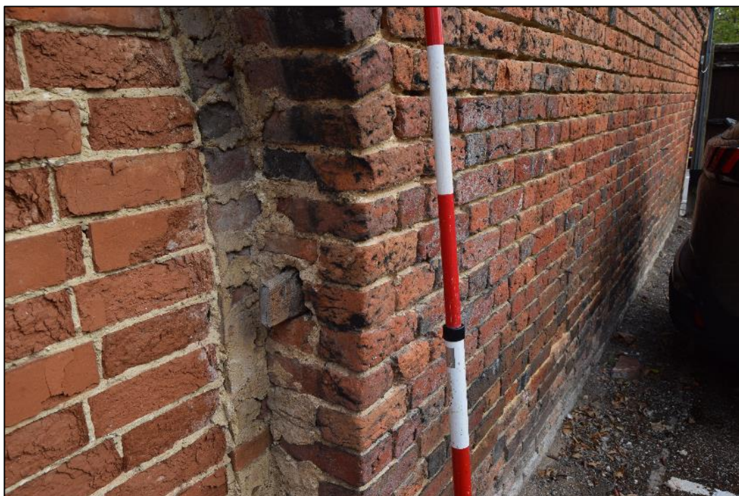
Plate 31: View looking NE towards the SE facing elevation of the wall, focusing of the right side of the infilled archway.
