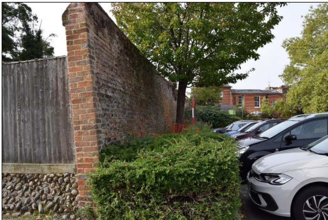
Plate 24: View looking SW along the NW facing elevation of the wall.
