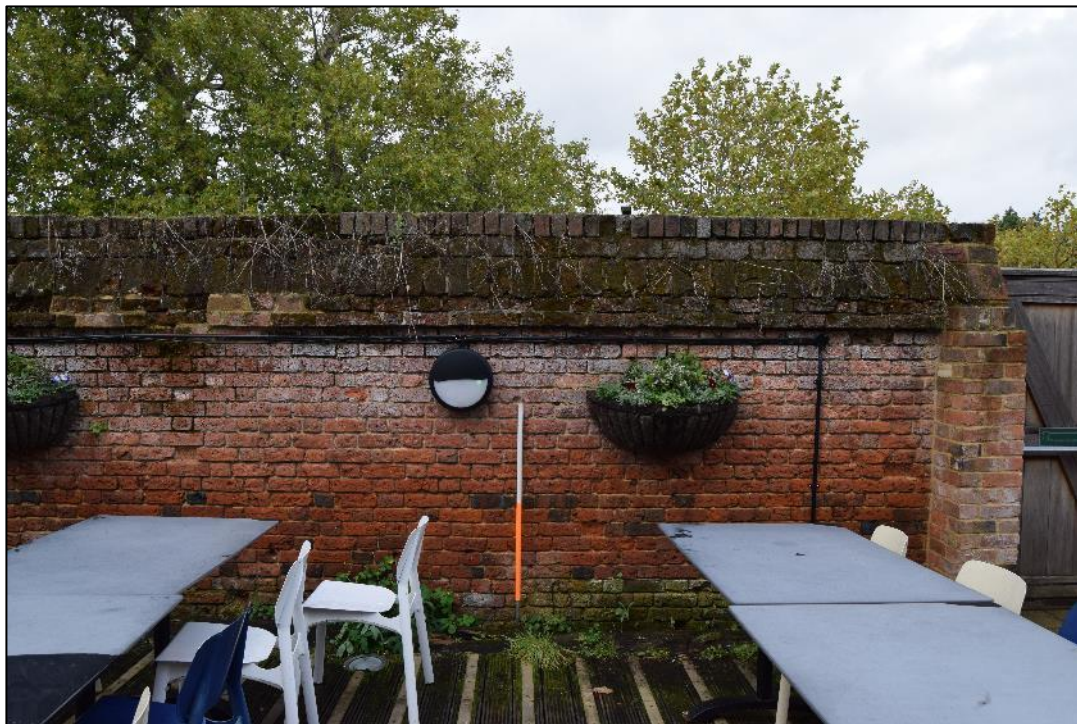
Plate 40: View looking NW towards the SE facing elevation of the wall.
