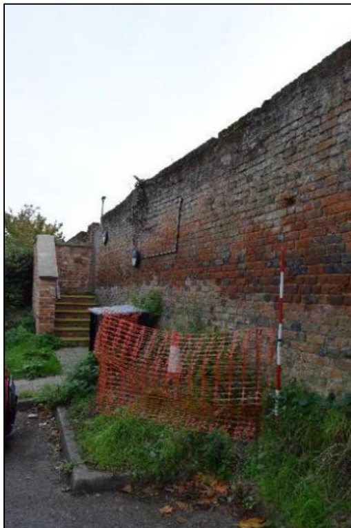
Plate 10: View looking NE along the NW facing elevation of the wall, towards the enclosed flight of steps.
