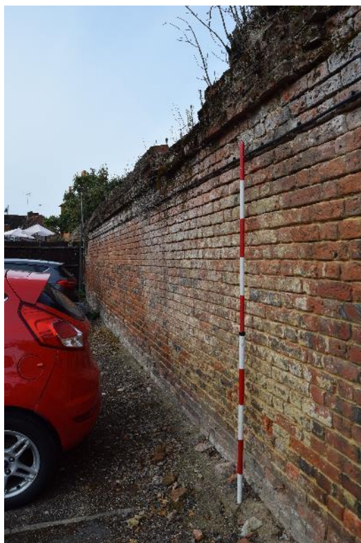
Plate 34: View looking SW along the SE facing elevation of the wall.
