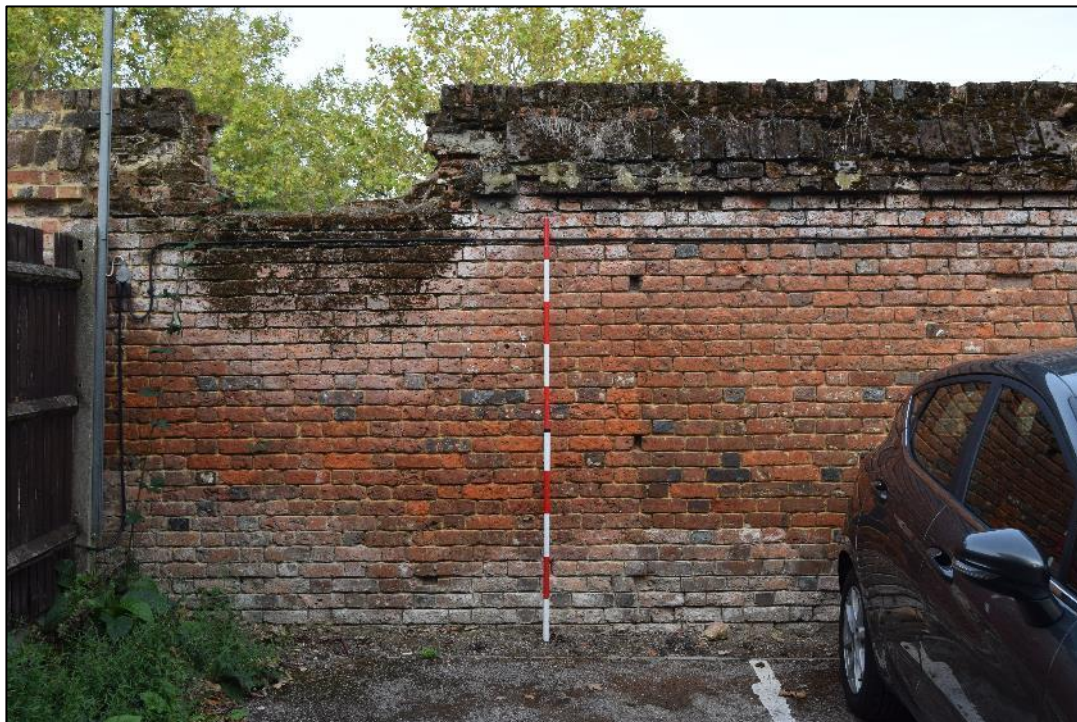
Plate 38: View looking NW towards the SE facing elevation of the wall.
