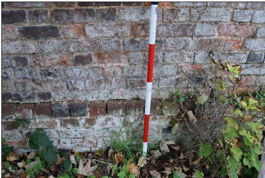
Plate 7: View of the foundation plinth to the NW facing elevation.
