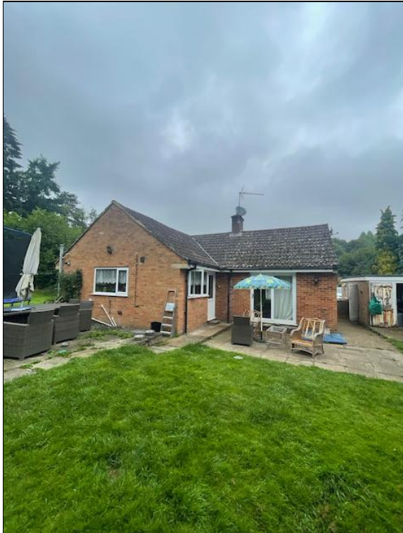
Photograph 9: Rear elevation with adjacent patio.
