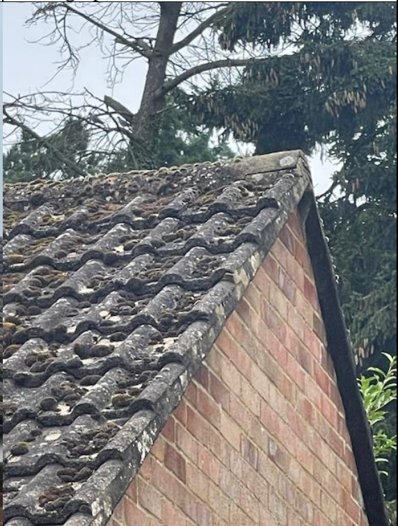
Photograph 4: Interlocking concrete roof tiles with no gaps.
