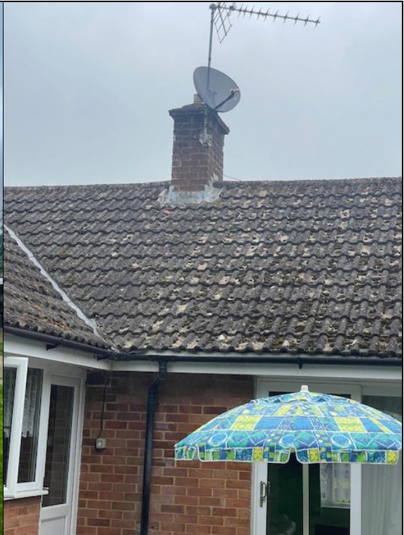
Photograph 10: Interlocking roof tiles with no gaps on rear elevation.
