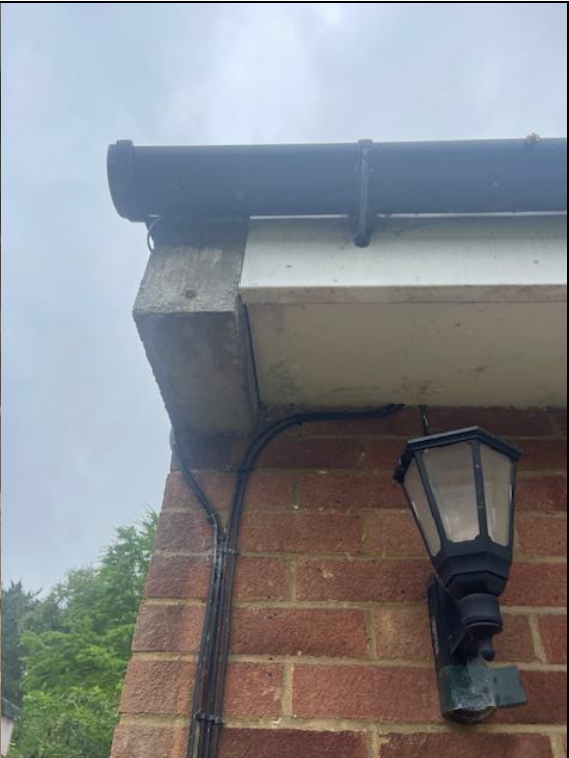
Photograph 6: Wooden soffits in good condition.
