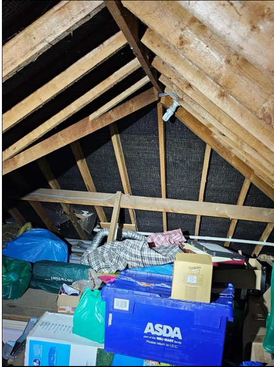
Photograph 25: Loft space used for storage.
