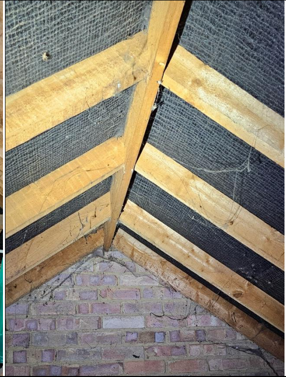
Photograph 26: Loft space, bitumen liner.
