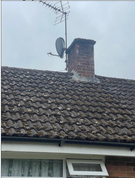
Photograph 3: Interlocking concrete roof tiles with no gaps.
