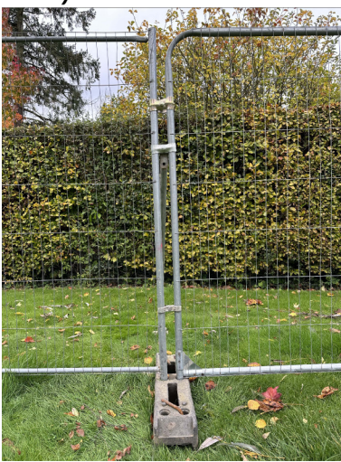
Protective Barrier (P.B.) (S.T.P.) Each panel will be clamped to the next using Heras anti-tamper couplers.
