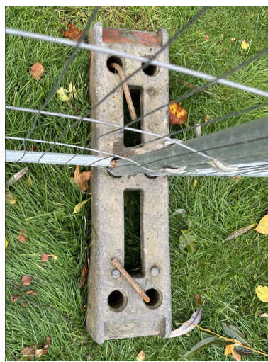
Protective Barrier (P.B.) (S.T.P.) Heras fencing panels, placed in rubber feet, which will be pinned to the ground using a soil pin. For impenetrable ground, the stabilisation bars will be mounted on a block tray and suitably weighted.
