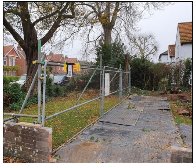
GP2: Tree protection barriers & trackmat ground protection
